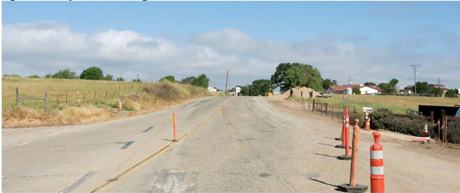
Figure 2-15 Key View 5—Existing Conditions
