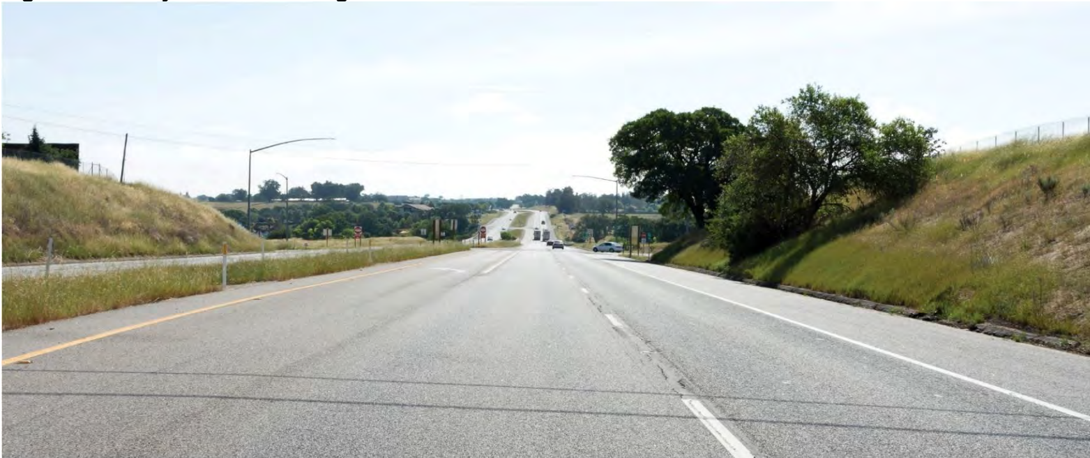
Figure 2-12 Key View 2—Existing Conditions
