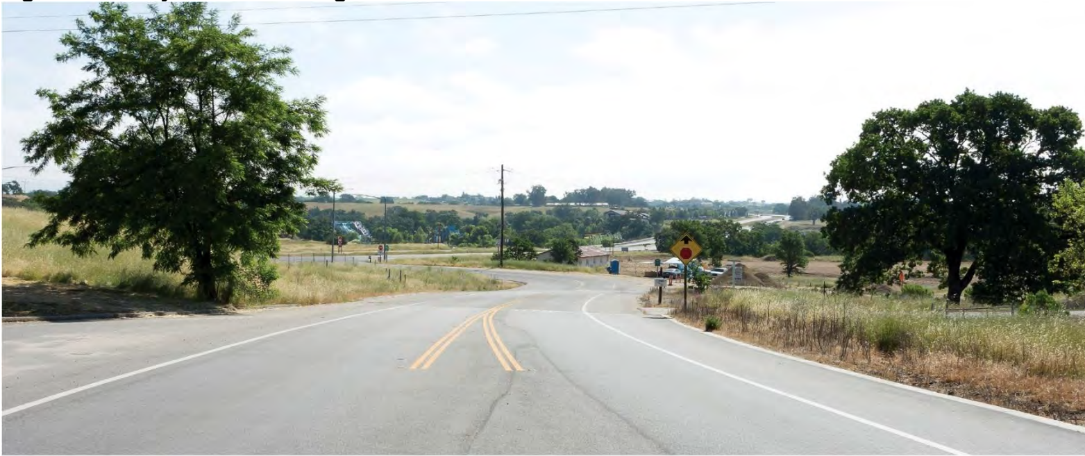
Figure 2-14 Key View 4—Existing Conditions
