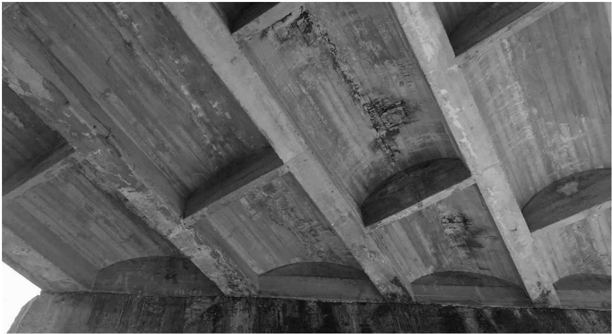
Underside of the bridge showing the jack arch construction.
