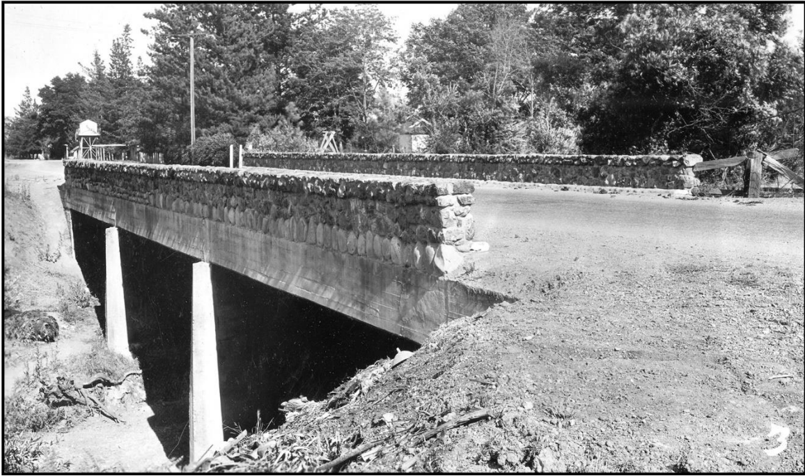
Photograph of the Alamo Pintado Creek Bridge, 1932. The bridge is a concrete-encased “jack arch” steel-stringer bridge with rustic stone masonry rails.
