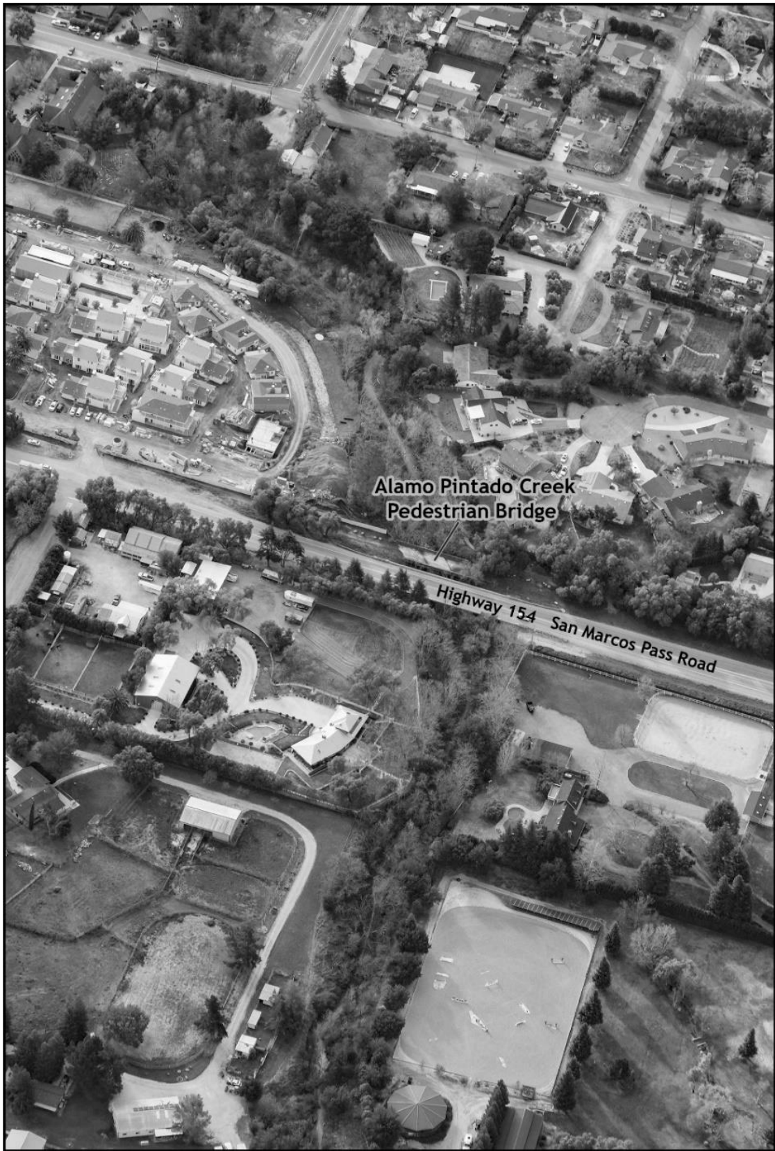
Aerial view facing south of a portion of the community of Los Olivos showing the Alamo Pintado Bridge along Highway 154.
