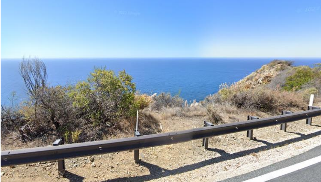
Figure 1-4 Stained Midwest Guardrail System
