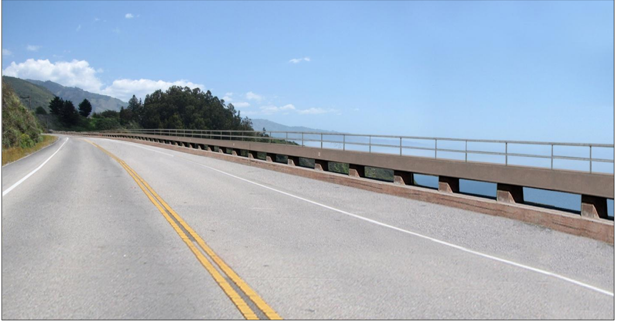
Figure 1-5 Concrete Open-Style Bridge Rail with Bicycle Rail
