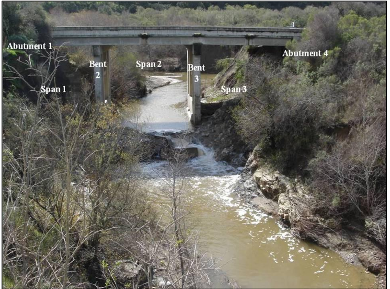
Figure 1-3 Bridge Elements
