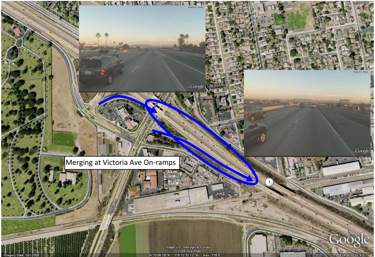
Figure 22 Southbound US-101 at Victoria Avenue On-ramps
