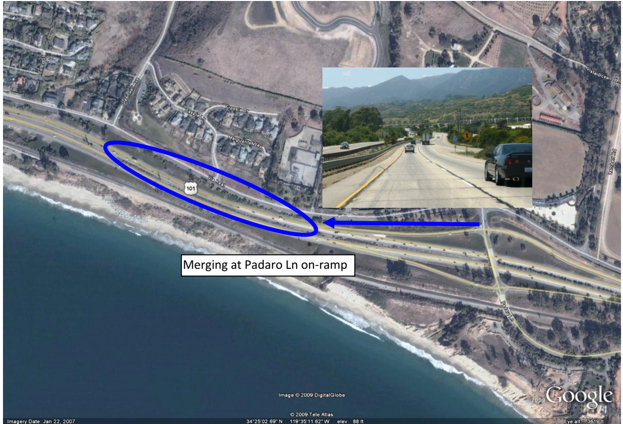
Figure 3 Northbound US-101 at Padaro Lane On-ramp
