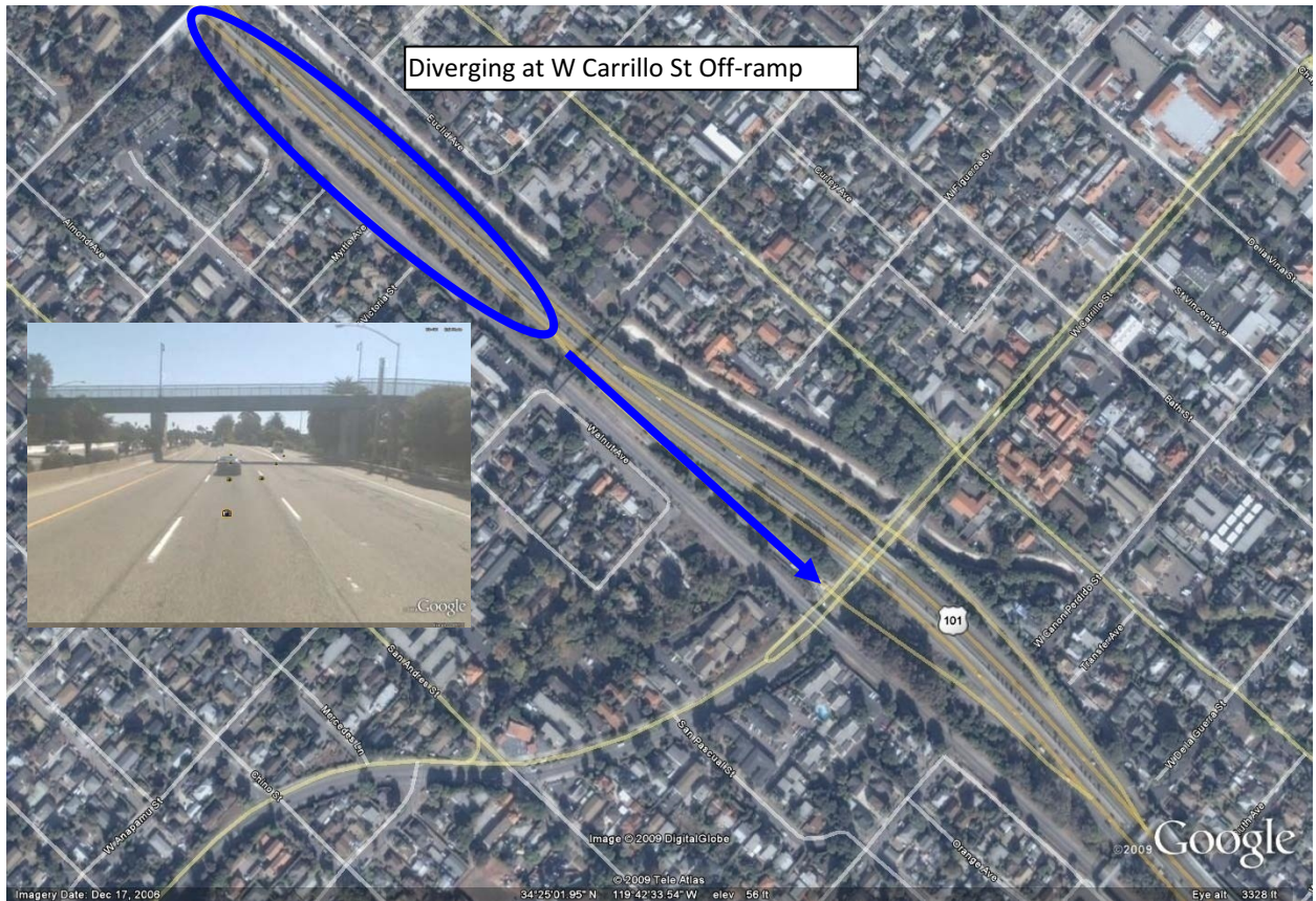
Figure 6 Southbound US-101 at W Carrillo Street Off-ramp
