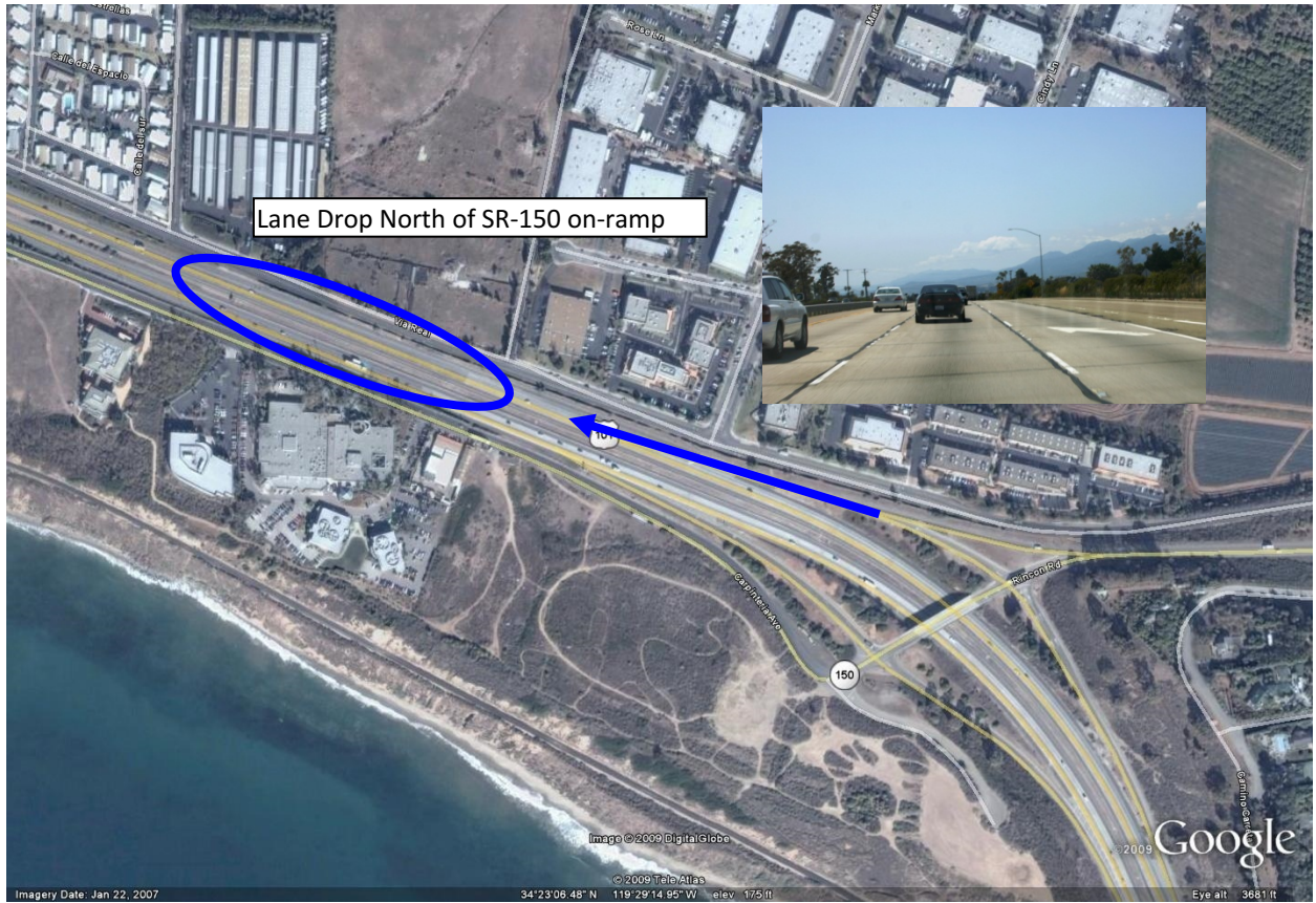
Figure 5 Northbound US-101 at Lane Drop North of SR-150 On-ramp
