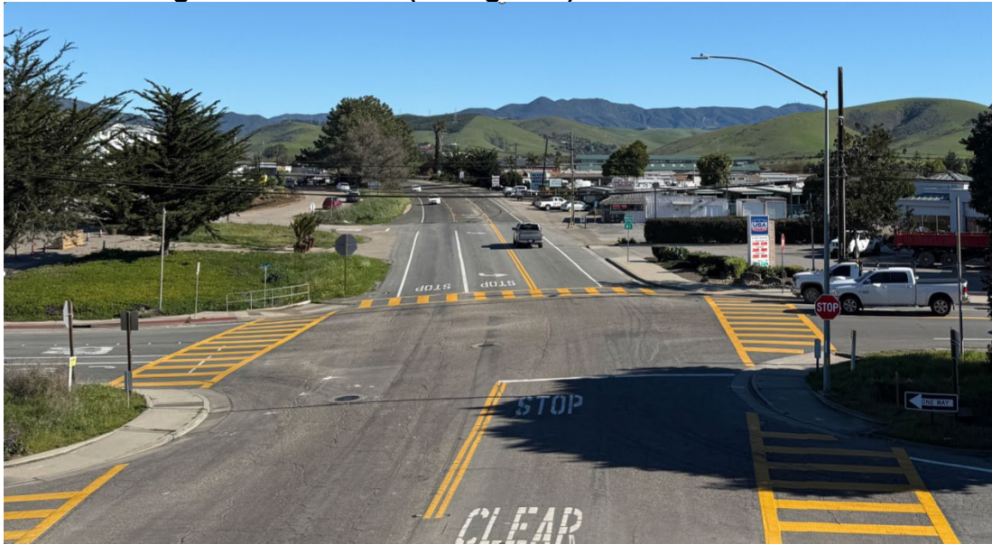
Figure 2.5 Existing Project Site View from State Route 1 Bridge Overcrossing State Route 41 (facing east)
