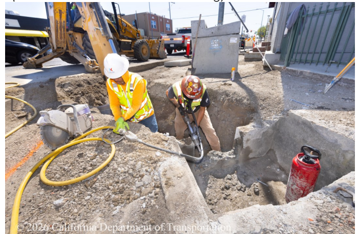
(Below: Crew due some deconstructing)
