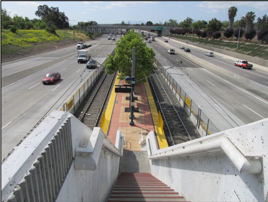
Figure 15. Light rail station in SR 87 median at West Virginia Street.
