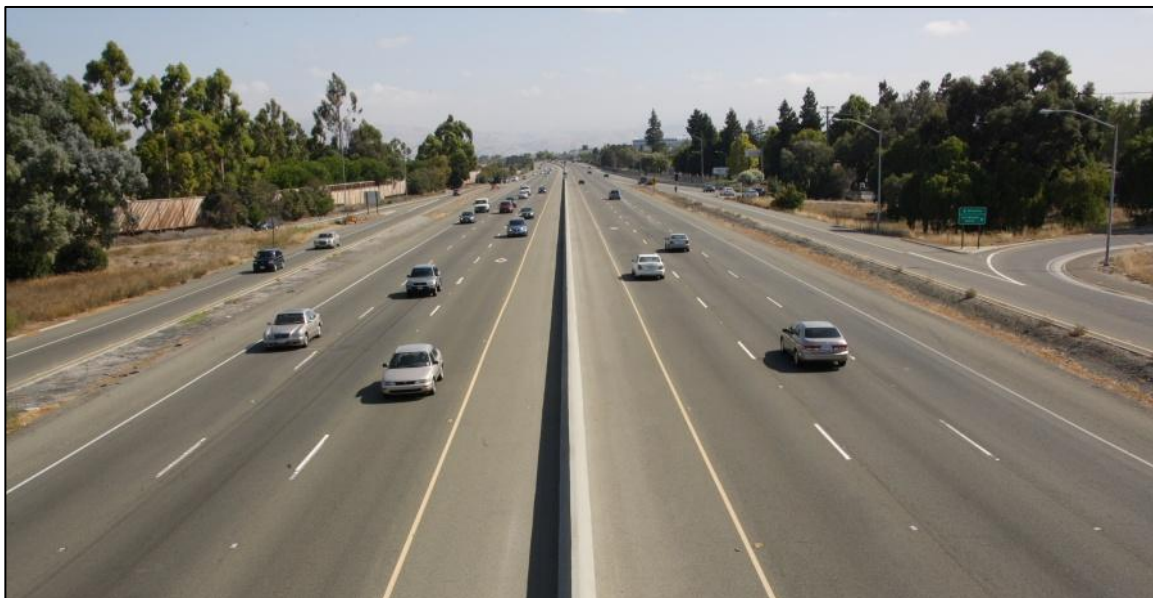
Figure 21. View from the Lawrence Expressway Bridge crossing SR 237.
