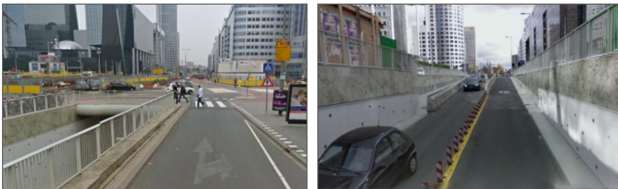
Figures 15a and 15b. European example of potential express lane infrastructure passing underneath an intersection; view at ground level to the left, view from roadway to the right.
