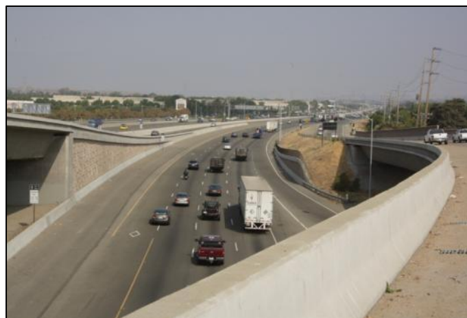
Figure 13b. View north to I-880; see view locator in Figure 11a. Source: D4 Caltrans Photography
