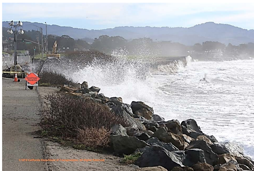
Surfers Beach erosion, Half Moon Bay
