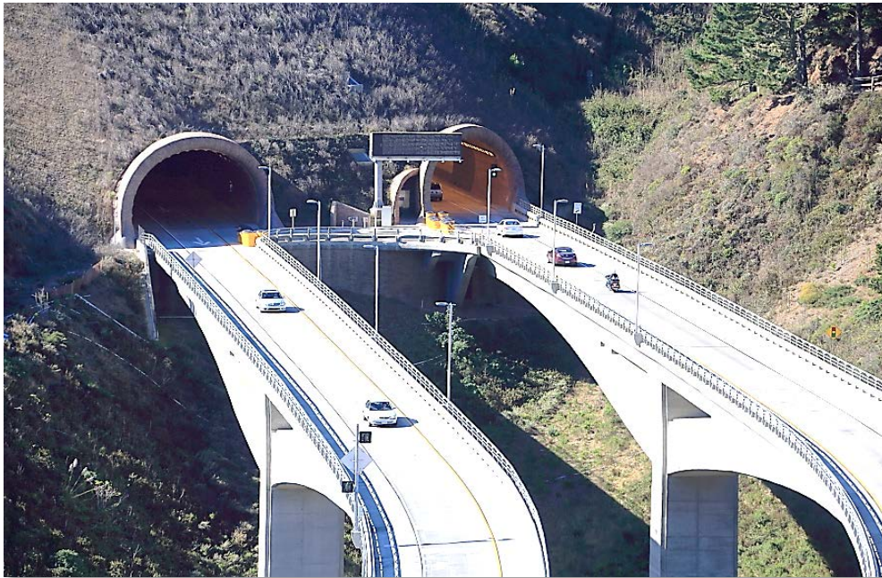
Tom Lantos Tunnels, south of Pacifica
