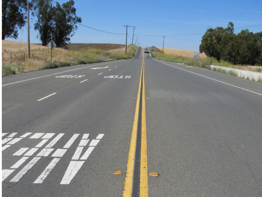
SR 113 looking north from junction with SR 12
