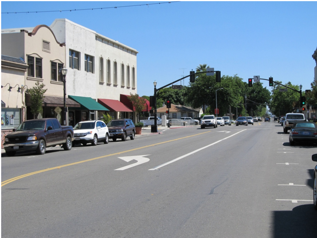
Segment B --Northbound SR 113 at A Street, Dixon
