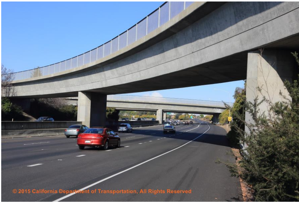
Union Pacific Rail Bridges over I-580 in southeast Richmond
