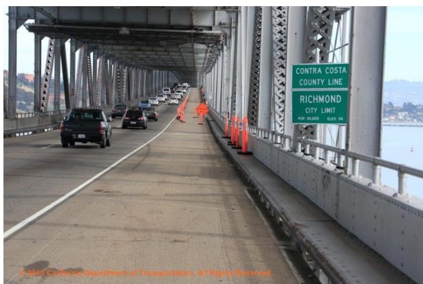
Existing Lower Deck of the RSR Bridge
