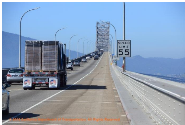
Existing Upper Deck
