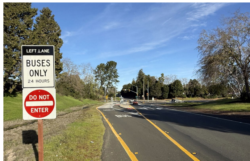
Bus only lane near the Imola Park and Ride in Napa. Source: Caltrans.
