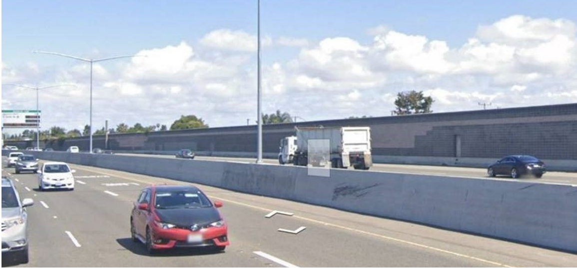
Figure 1-5. Example Concrete Barrier Type 60M with Optional Lighting Attached
