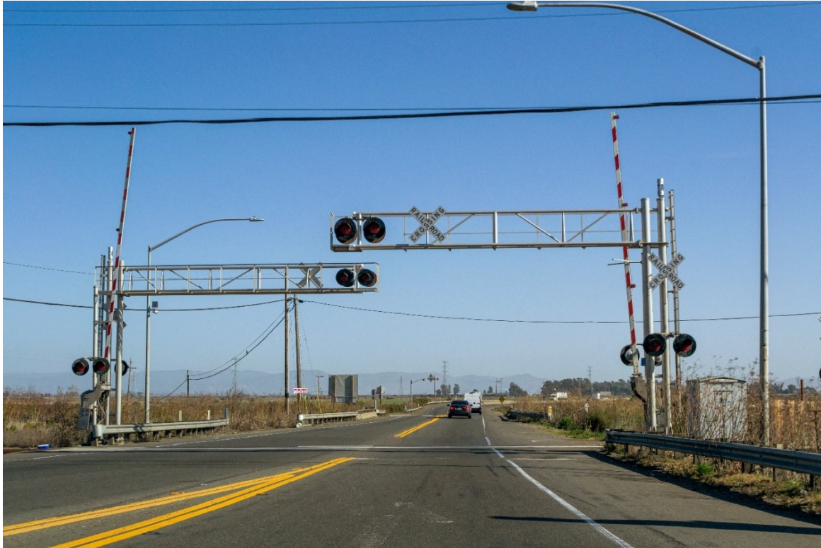
Figure A-8. KV 1 (Eastbound SR 37 Looking East) Existing Conditions
