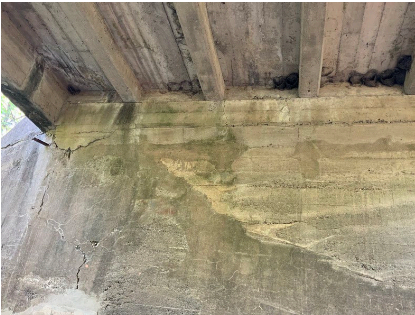
Photo 3: Looking westbound at Abutment 1 displaying the spall at the bottom face of Girder 2 (taken April 2021).
