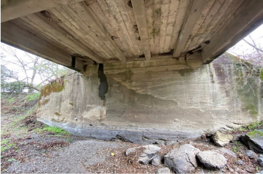
Photo 2: Looking westbound at Abutment 1 displaying patched and repaired concrete areas (taken in 2015).
