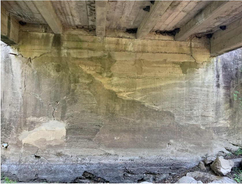
Photo 4: Looking westbound at Abutment 1 displaying multiple spalls in the face; Girder 2 (left), Girder 1 (right) (taken April 2021).
