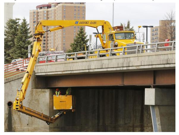
Figure 2-2 Example of an Under Bridge Inspection and Utility Truck
