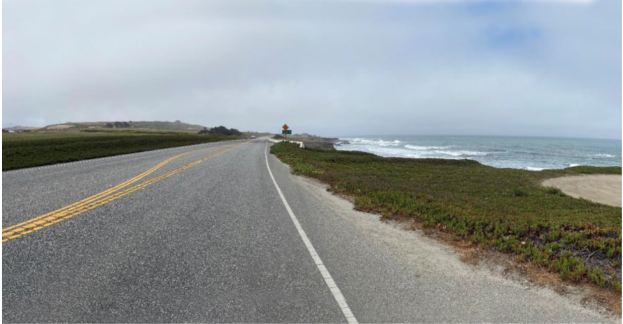
Figure 2-4. Representative View from Southbound SR 1 Approaching the start of the Eastward Roadway Realignment
