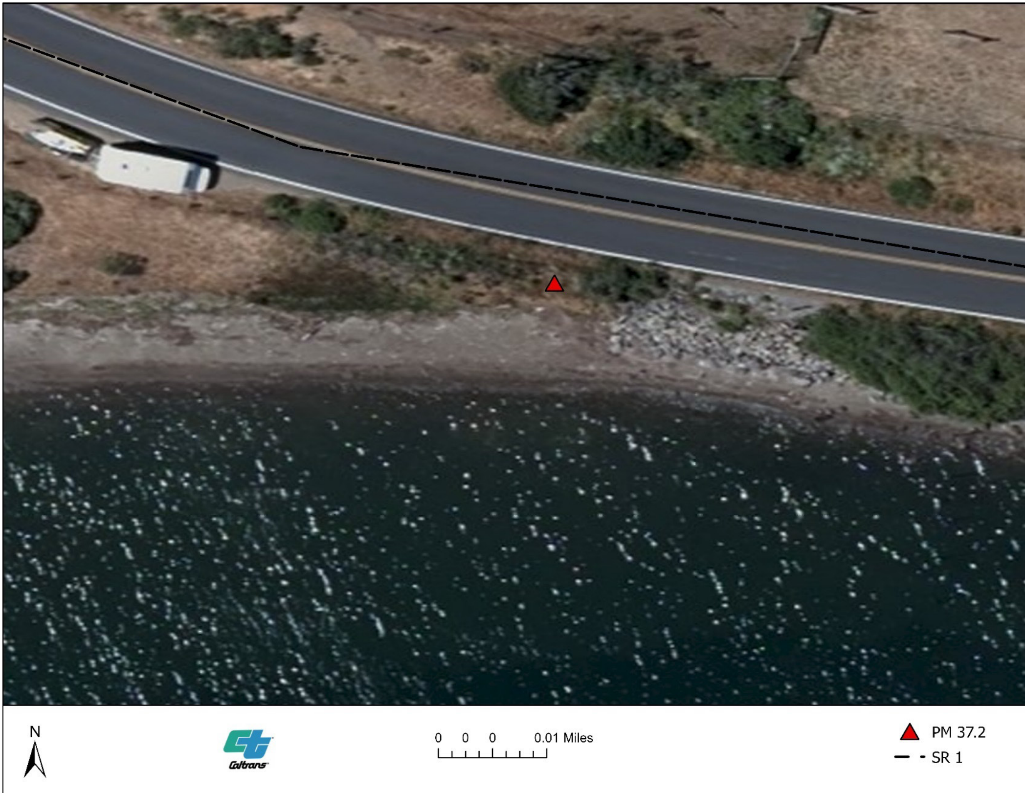
Figure 4. Aerial photo of existing conditions.
