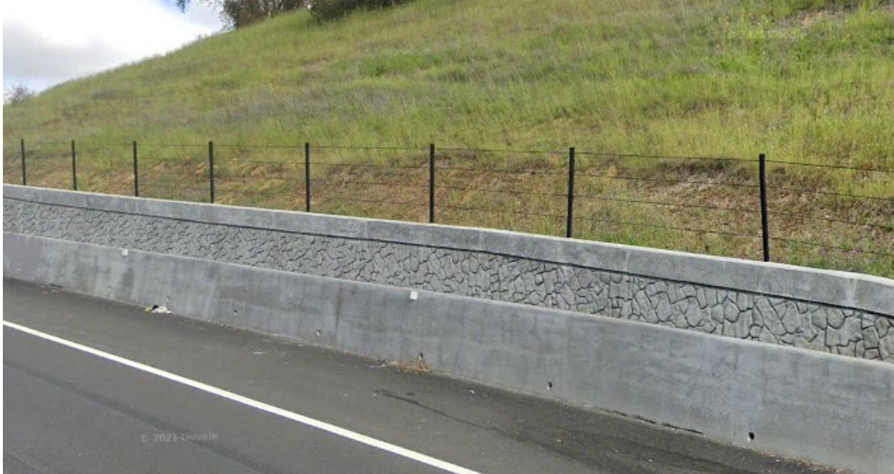
Figure 2.6-1. Retaining Wall Topped by Cable Barrier along Existing Northbound On-ramp to I-680 from Sunol Boulevard
