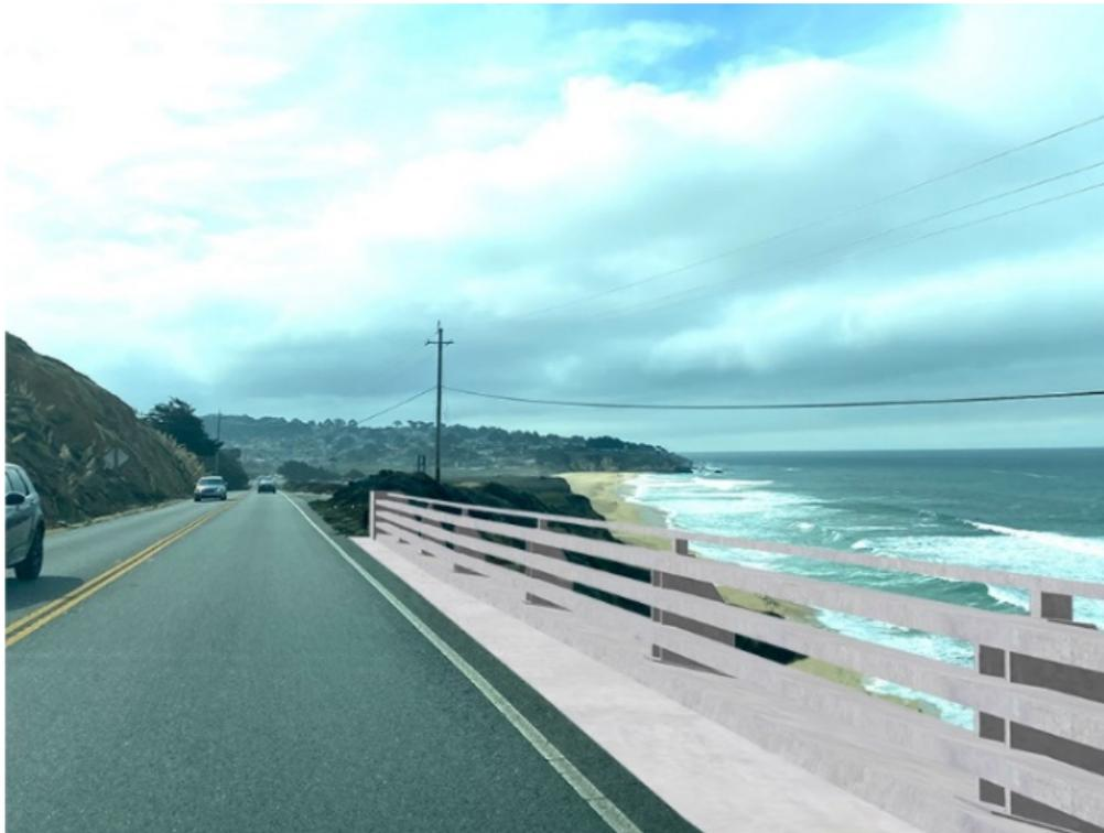
Build Alternative 1 with Steel Barrier ST-75
