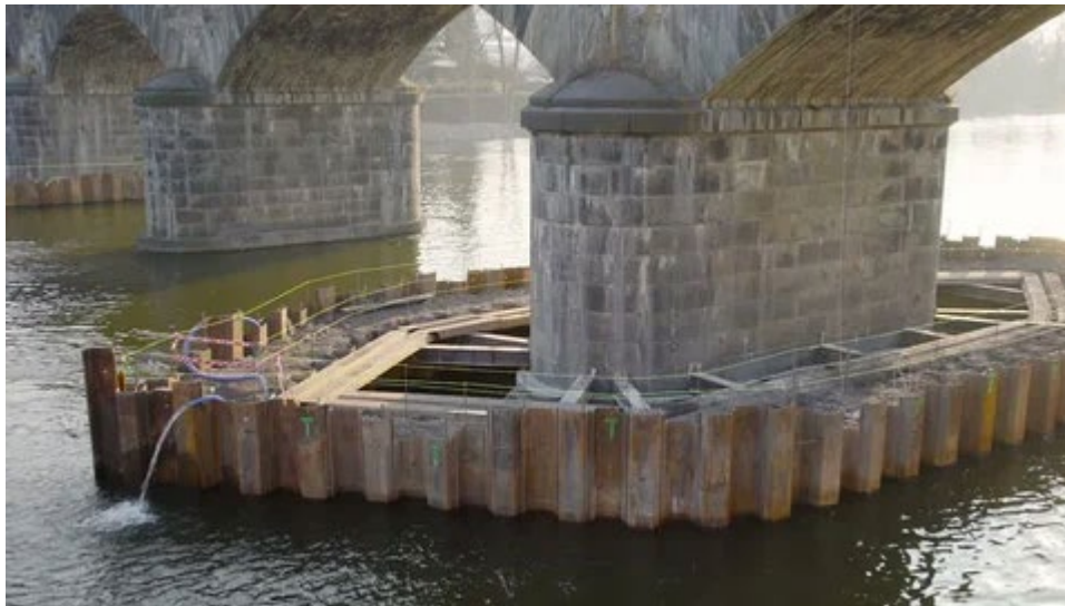
Figure 1-7: Example Cofferdam around Bridge Foundation
