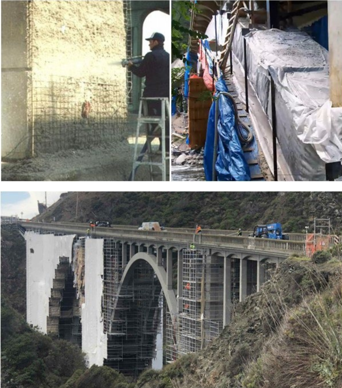
Figure 1-5: Example of Electrochemical Chloride Extraction Set-Up
