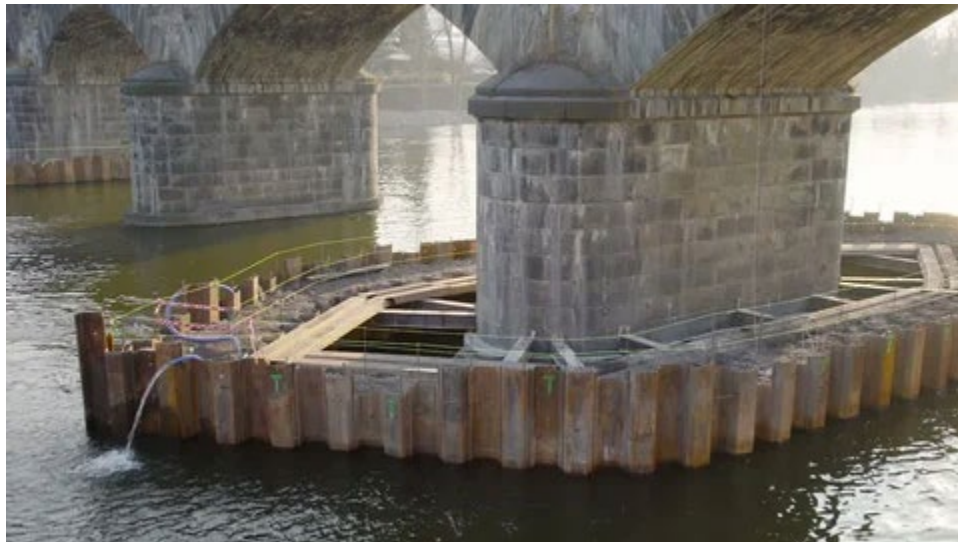
Figure 1-7: Example Cofferdam around Bridge Foundation
