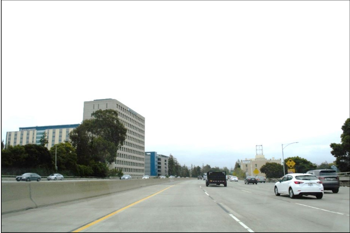
Figure 2.1-8. Photo of VAU 1 from EB I-580
