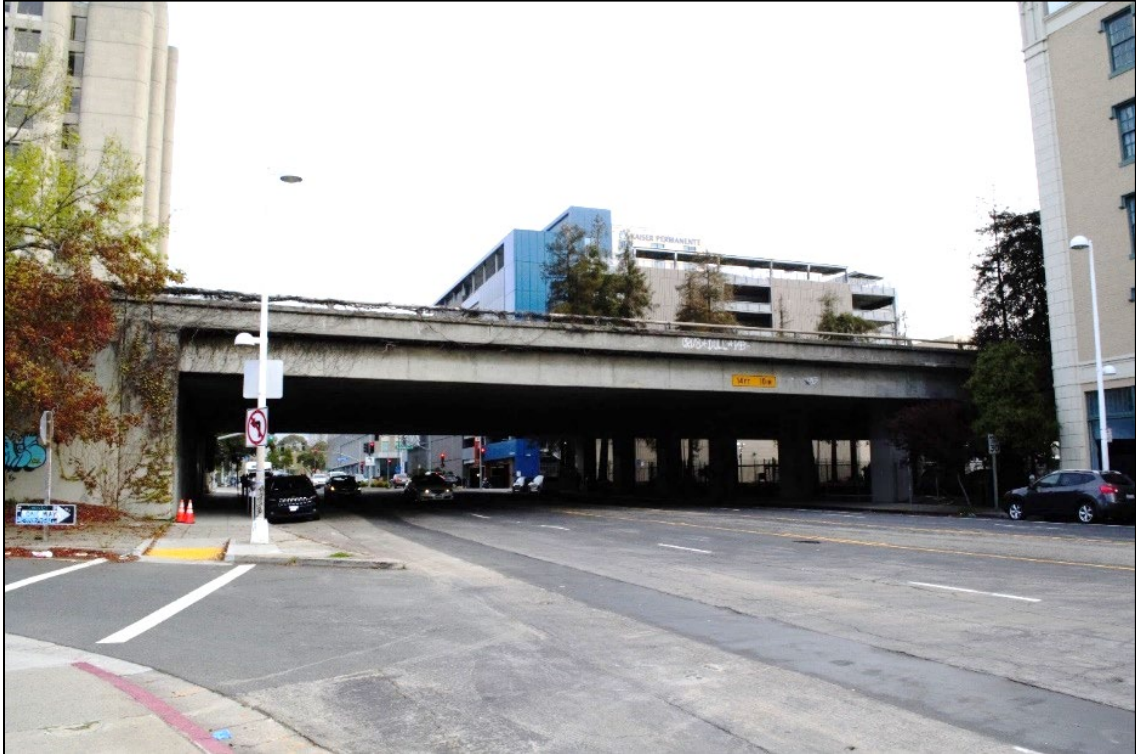
Figure 2.1-9. Photo of VAU 1 from Broadway Avenue
