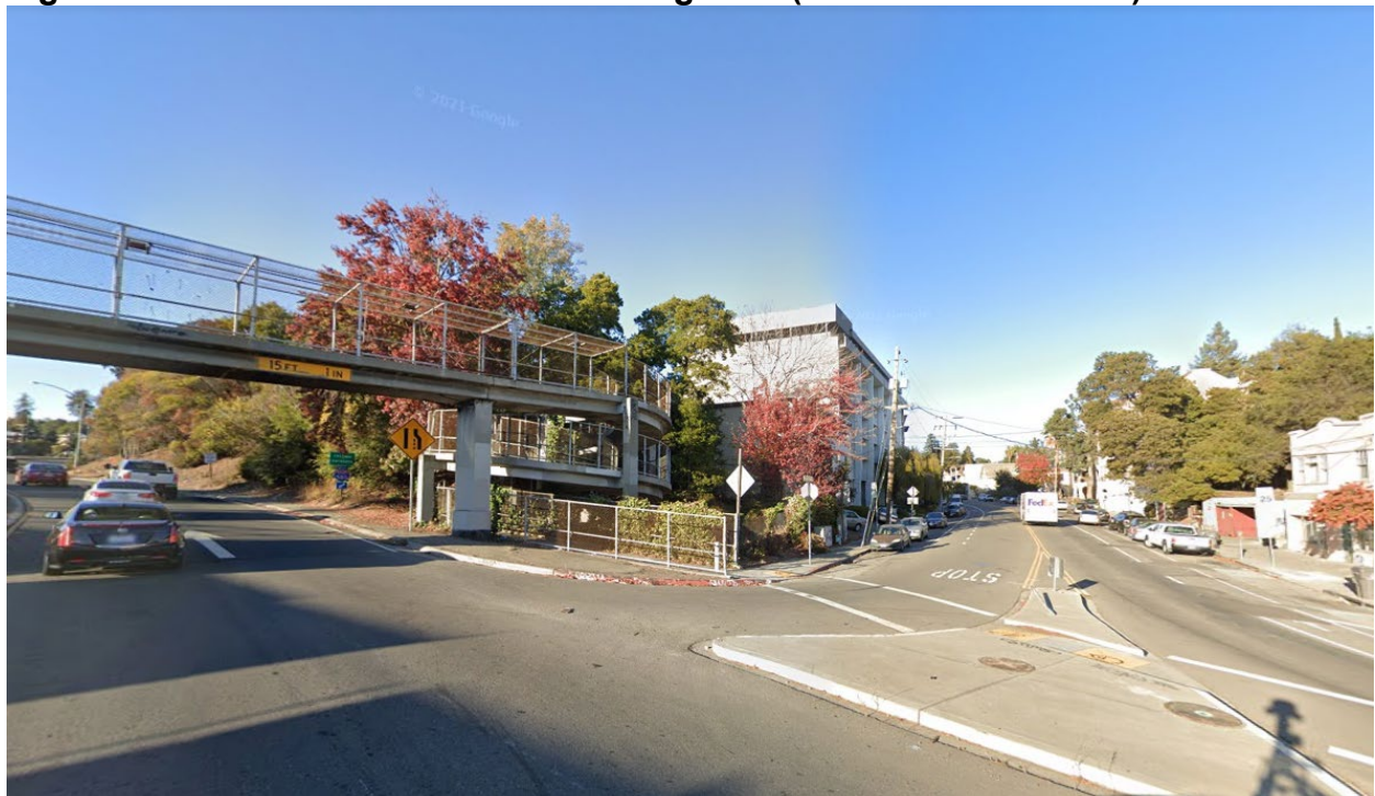
Figure 1.3-5. View of East End of Existing POC (Santa Clara Avenue)
