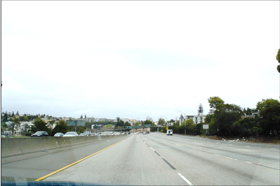
Figure 2.1-10. Photo of VAU 2 from EB I-580
