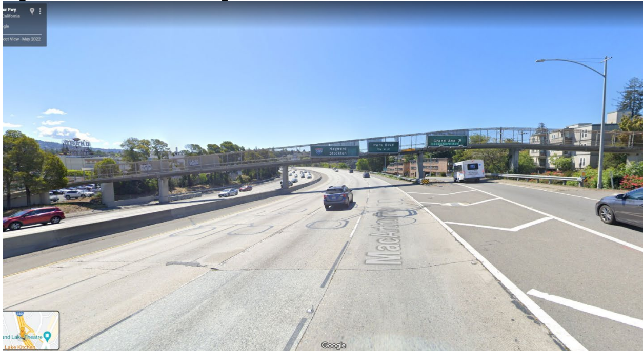
Figure 1.3-4. View of Existing POC from Eastbound I-580
