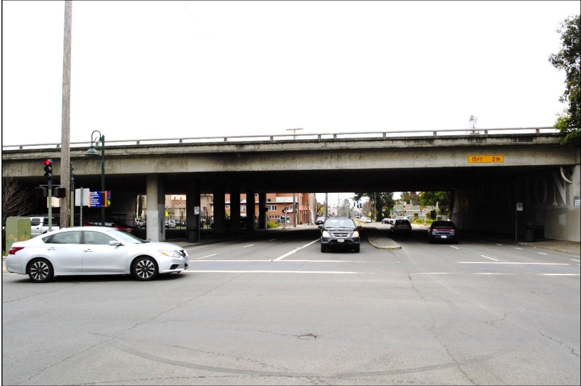
Figure 2.1-12. Photo of VAU 3 from Fruitvale Avenue
