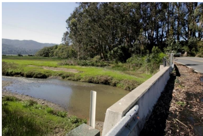
Figure 2. Culverted Creek at Millerton
