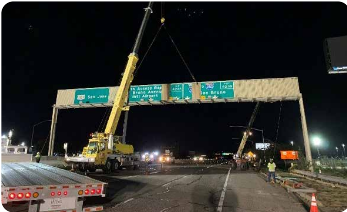
Construction crews removing an existing overhead sign structure on U.S. 101.
