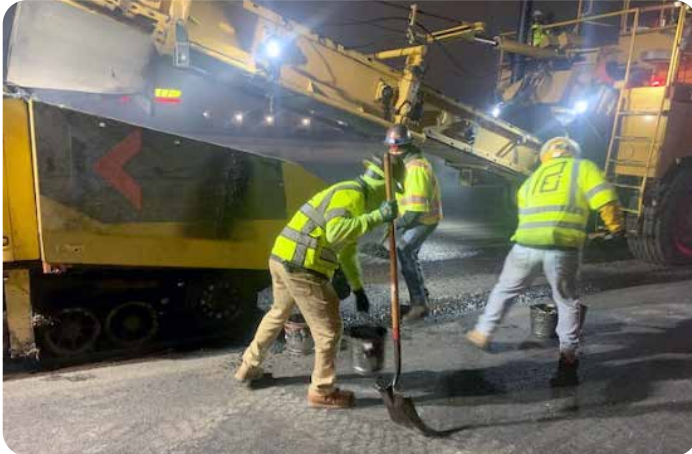
Construction crews repaving the freeway lanes north of Broadway.
