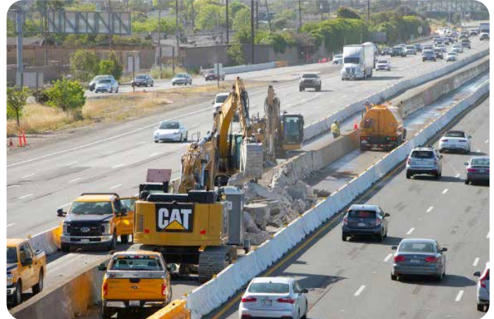
Construction crews demolishing the median barrier.
