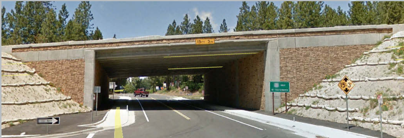
Example: Sly Park Road Undercrossing - Looking North
