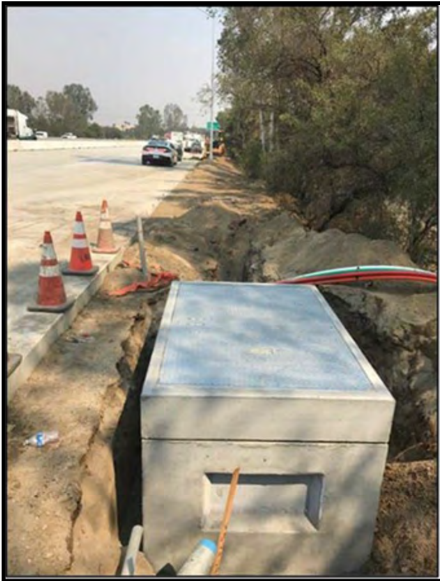
Figure 5. Vault Installation
