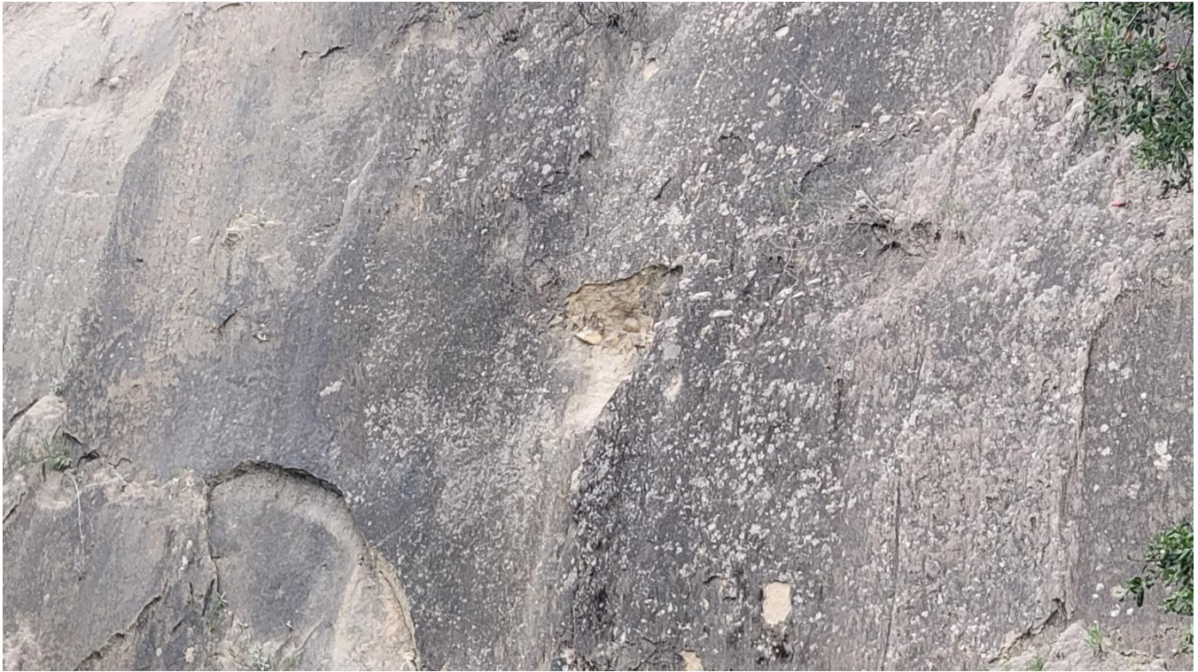
Figure 4. Tsn deposits, close up, EB SR-74 ROW approx. 125-ft east of drainage feature (window survey, no scale). Location Sheet: Layout-17
