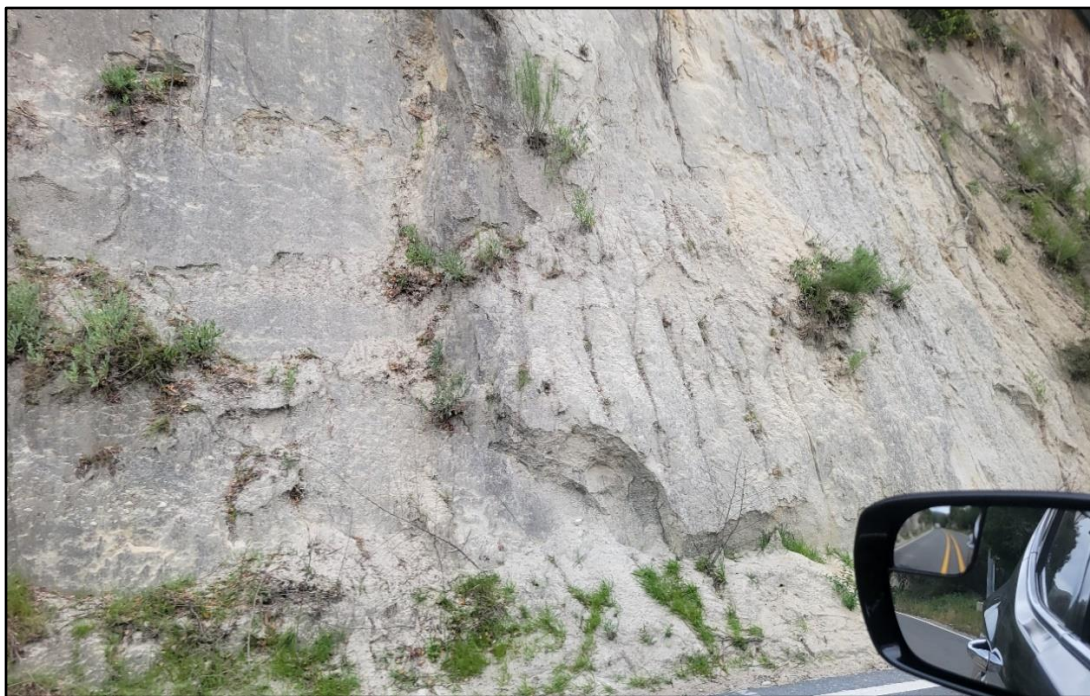
Figure 10. Tss Deposits, pavement rehabilitation work along WB SR 74 ROW, PM 5.4/5.5, view south.
