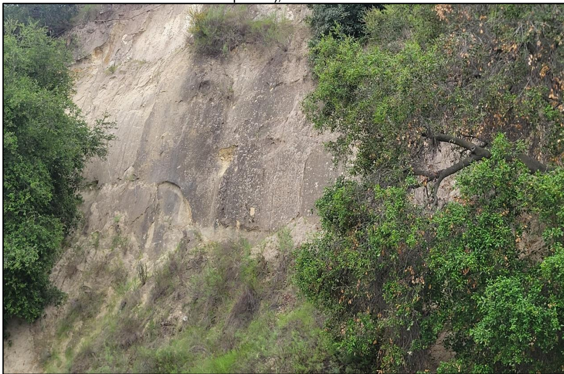
Figure 8. Proposed drainage location #2 Tss Deposits (~100 ft. east) along EB SR 74 ROW, PM 4.2/4.3, view south.
