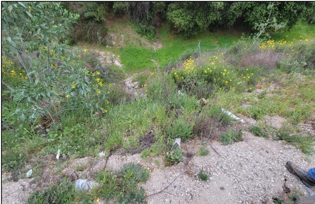
Figure 5. Proposed drainage location #2 along EB SR 74 ROW, PM 4.2/4.3 (Tss Deposits), view south.
