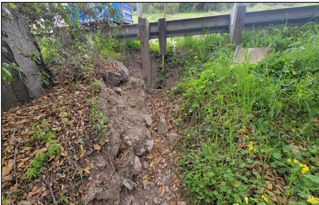
Figure 6. Proposed drainage location #1 along slope of EB SR 74, PM 5.2/5.3 (Qy/s deposits), view south.
