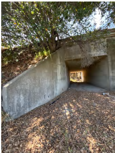
Photo 13: View of Feature 22 that is 12 ft concrete box culvert with an earthen drainage channel on either side of the culvert.
