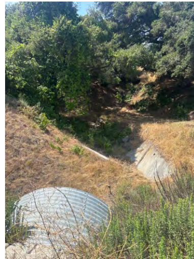
Photo 10: View of Feature 13 that is a concrete v-ditch that catches flows from a culvert.
