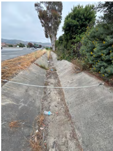
Photo 5: View of Feature 6 that is a concrete, trapezoidal drainage channel.
