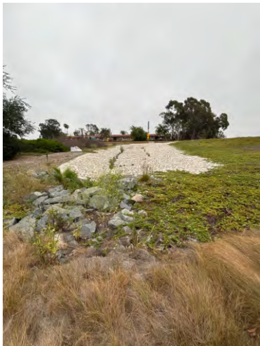
Photo 3: View of Feature 5 that is a concrete/cobble, shallow drainage channel.
