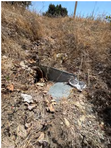
Photo 11: View of Feature 15 that is an earthen drainage channel that drains from a corrugated metal pipe culvert.
