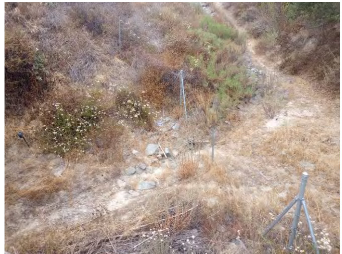
Photo 12: View of Feature 20 that is an earthen drainage channel that flows from an 8 x 8 ft concrete box culvert under SR-74.
