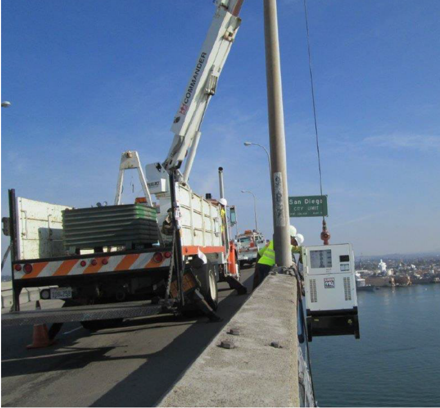
Figure 1-12 Simulated Horizontal Net Obstruction of Generator Access
