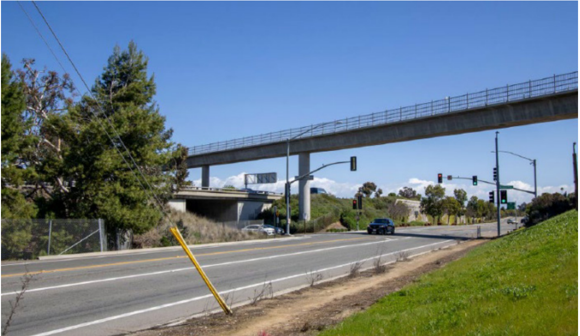
Figure 2-16: KV #6 – Existing Conditions
