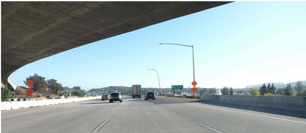
Figure 2-6: KV #1 – Existing Conditions
