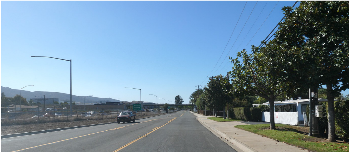
Figure 2-14: KV #5 – Existing Conditions
