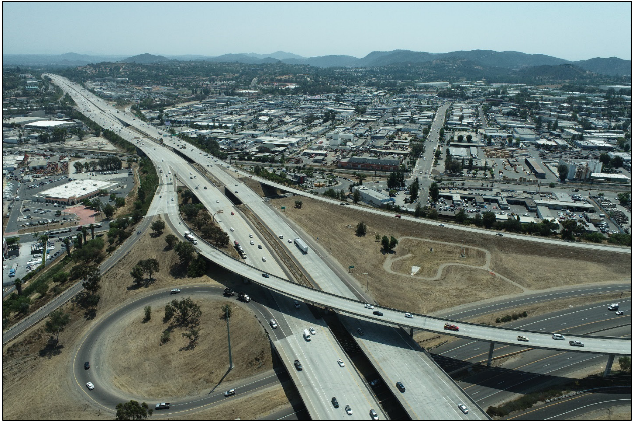
Figure 2-3: SR 78/I-15 Interchange VAU - Aerial View Looking South at I-15
