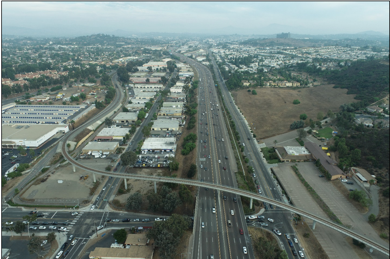
Figure 2-2: SR 78 Frontage Roads VAU - Barham Drive Aerial View at Woodland/Barham UC Looking East.
