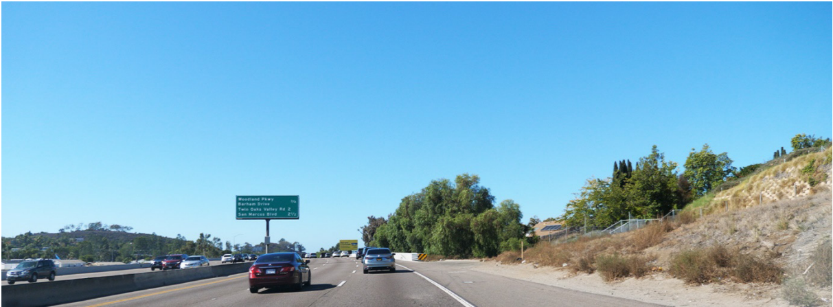
Figure 2-10: KV #3 – Existing Conditions
