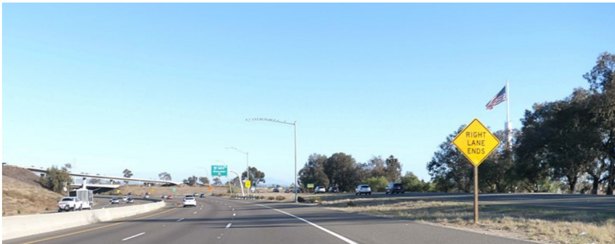
Figure 2-8: KV #2 – Existing Conditions
