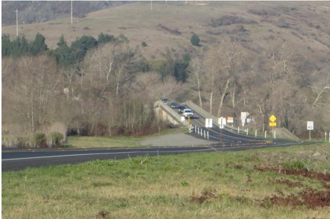
Traffic platoon forming on Fernbridge (PM 78.2)
