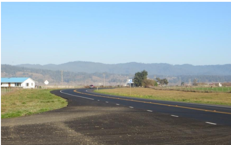
A typical section of Route 211 in the Lower Eel River Valley (PM75.8)
