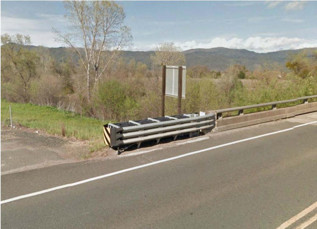
**Metal Beam Guardrail Transition Barrier**
