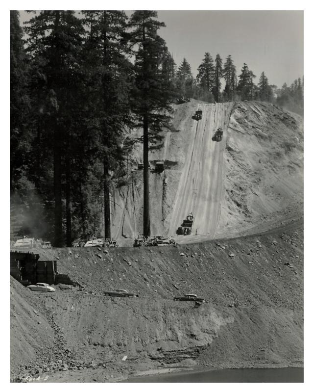
Figure 7. Representative photo of historic US 101 construction near Dyerville. Note the rerouted portion of the South Fork Eel River in the foreground. (State of California, Division of Highways, 1956)
