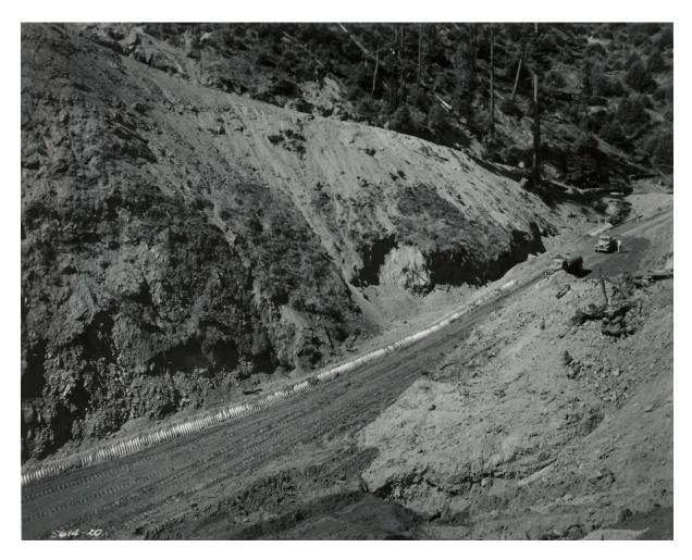
Figure 8. Representative photo of historic US 101 construction near Dyerville showing culvert installation. For scale, two trucks and a worker can be seen at the center of the right side of photo. (State of California, Division of Highways, 1956)
