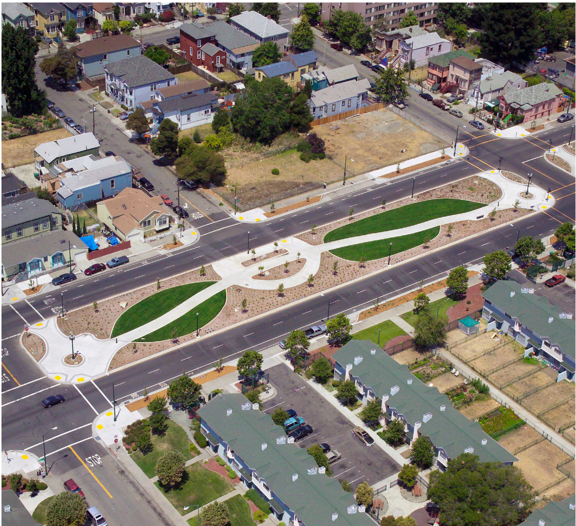
Photo 22: The new Mandela Parkway in Oakland, California, following conversion from the Cypress Street Viaduct.
