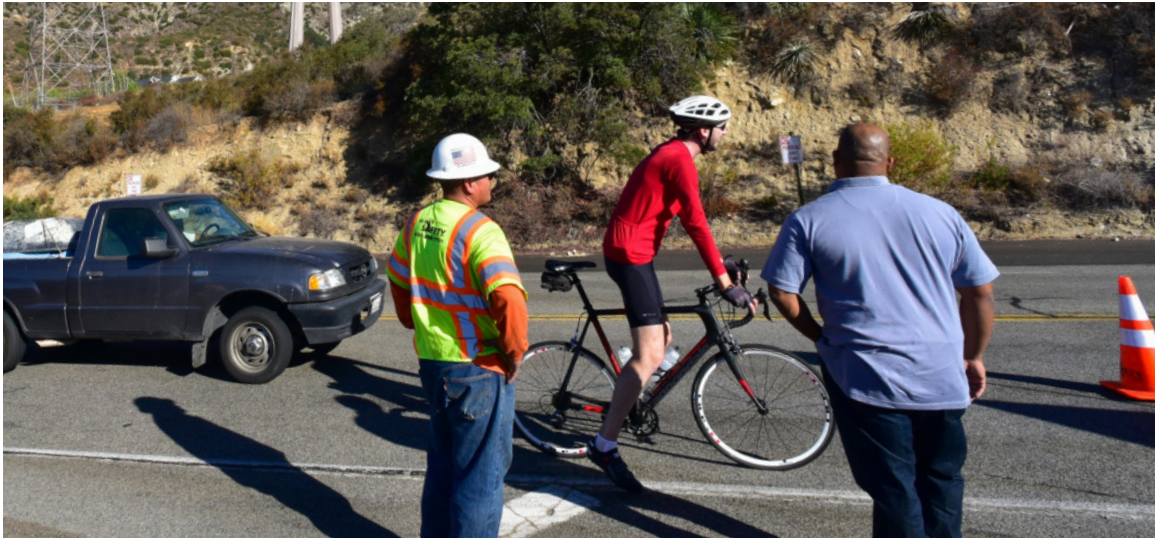
Photo 8: A few Caltrans workers run a bike consideration test on State Route 2.
