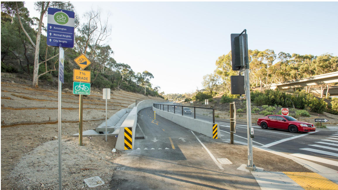
Photo 15: Commuter bike path with wayfinding signs.
