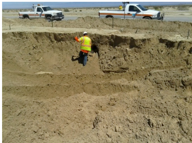
TWIN PIPES REPAIR WORK HIGHWAY 86
