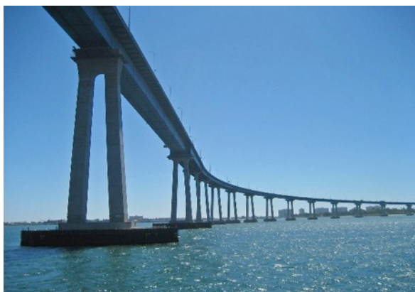
SAN DIEGO CORONADO BRIDGE
