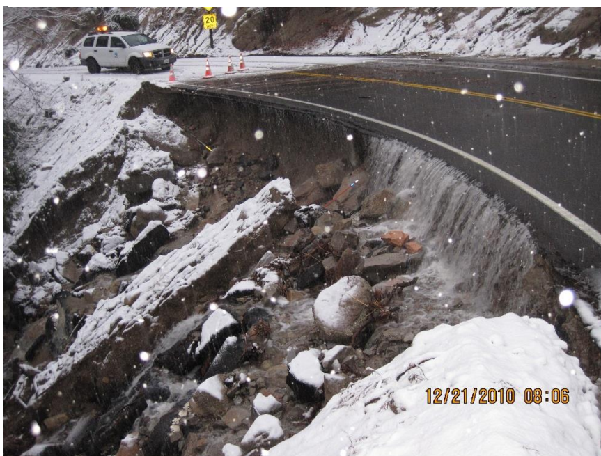
FIGURE 3: CULVERT OVERFLOW ON WILLOW CREEK ROAD
