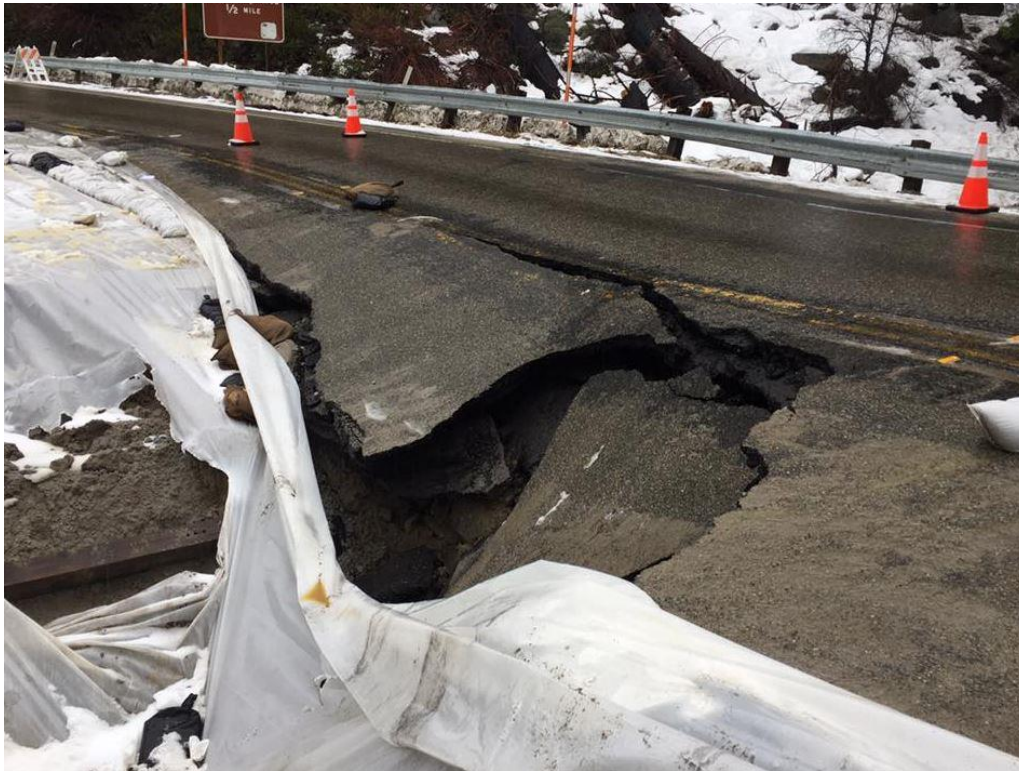
FIGURE 17: HIGHWAY 41 WASHOUT
