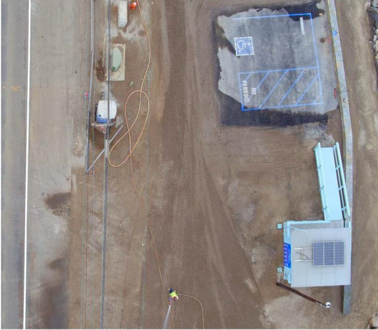
6/15/2016 New ADA compliant parking space.
