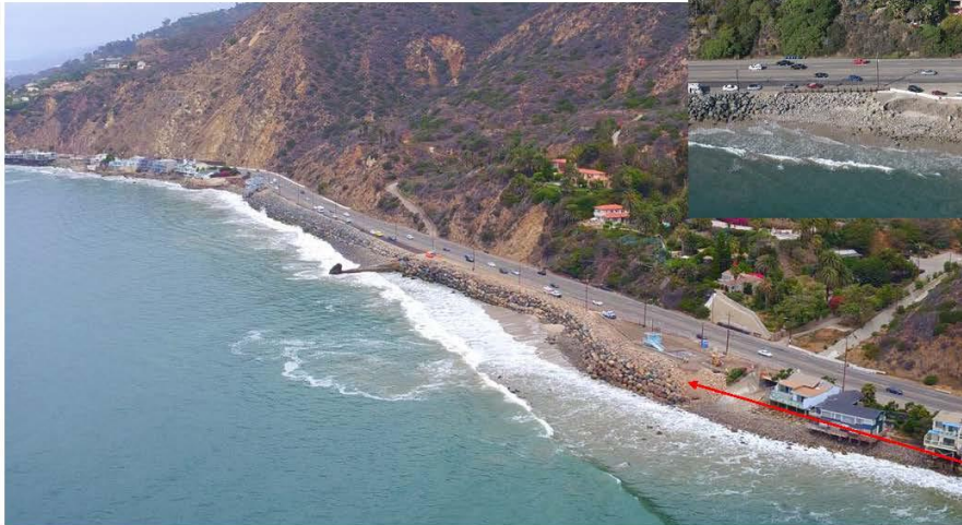
6/15/2016 Aerial of completed project looking north.
