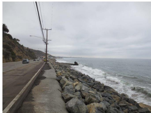
6/15/2016 After photo looking southbound.
