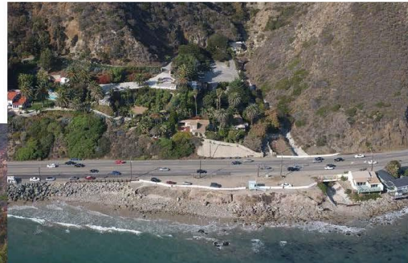
10/1/2004 Aerial of project location looking east at lifeguard tower.
