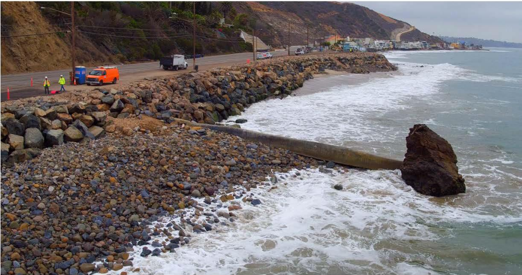
6/15/2016 Aerial of southbound completed project just west of beach access #3.
