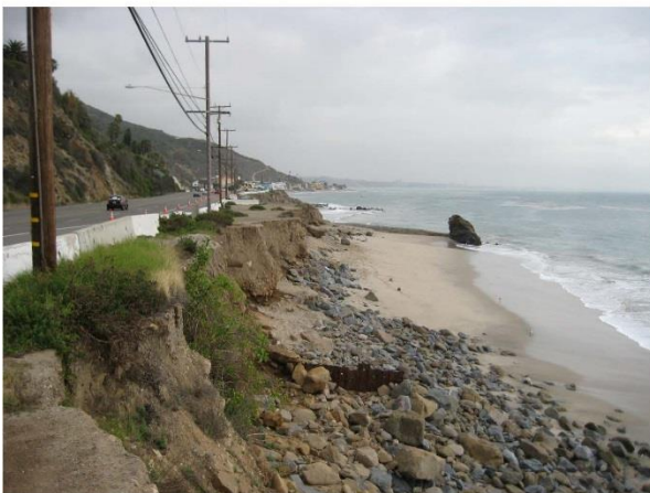
6/15/2016 Before photo looking southbound.
