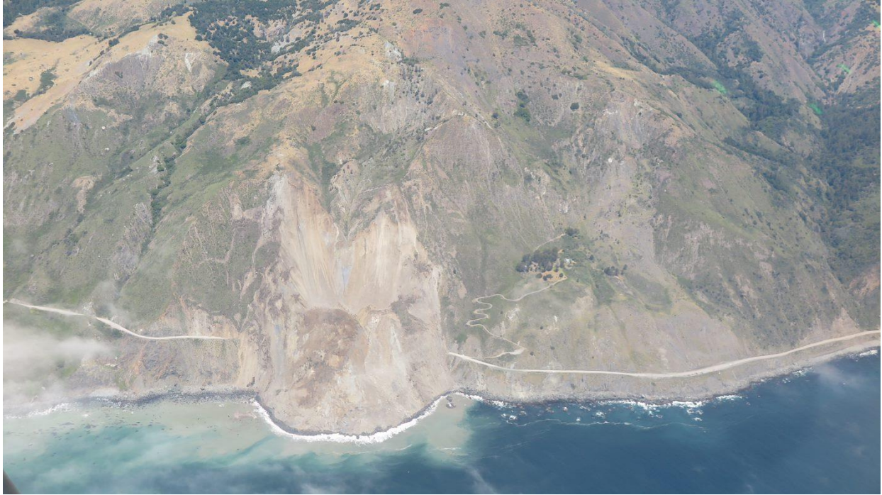
FIGURE 32: MUD CREEK SLIDE AND AFTER
