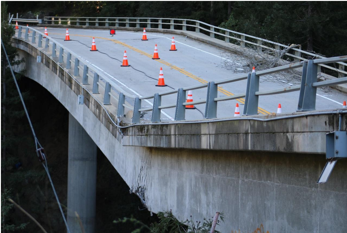
FIGURE 31: PFEIFFER CANYON BRIDGE BEFORE AND AFTER
