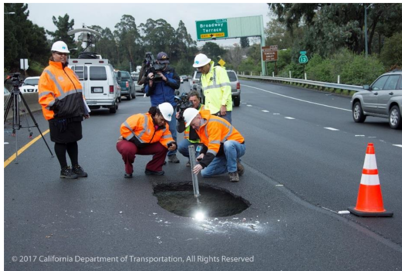
FIGURE 2: SINKHOLE ON HIGHWAY 13
