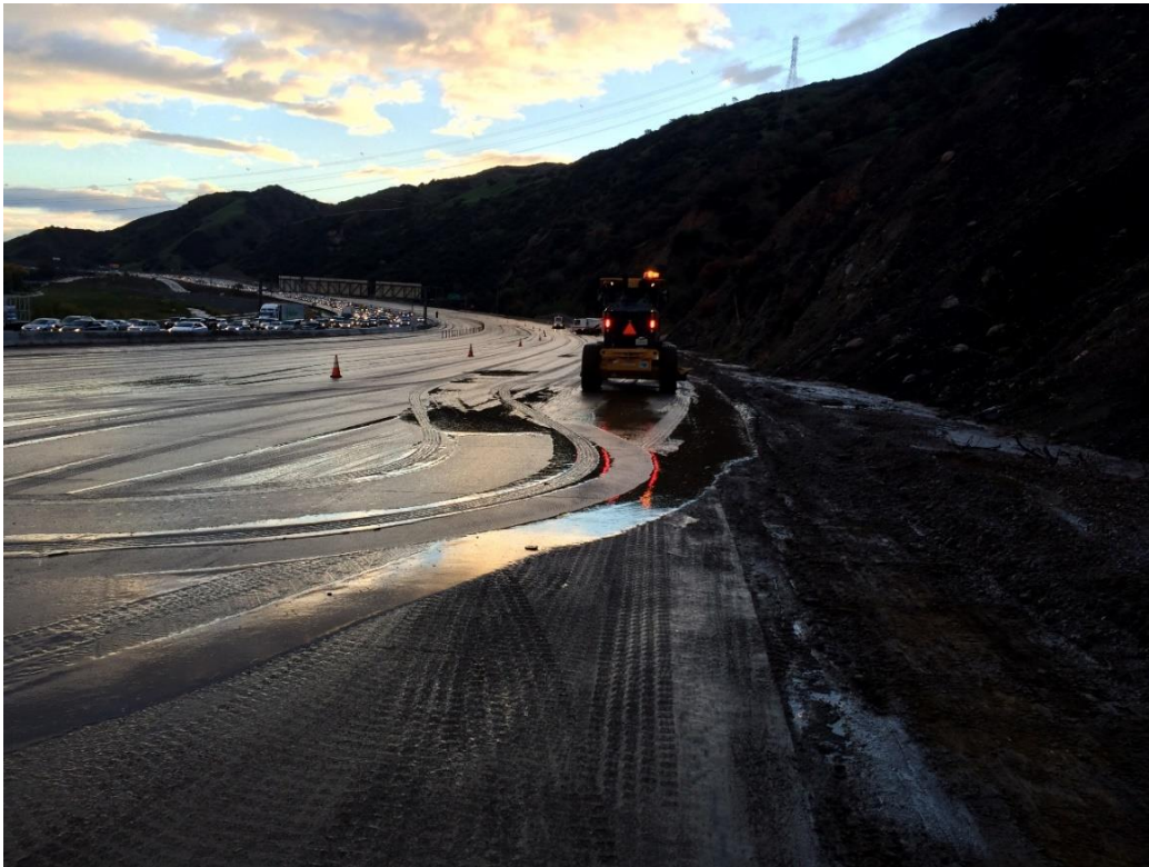
FIGURE 3: TRAFFIC DISRUPTION FROM ROCKSLIDE ON SR 91
