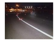
Enhancement "B" was the installation of rows of one and two-way red retro-reflective pavement markers in a closely-spaced pattern near the end of the exit ramp.
