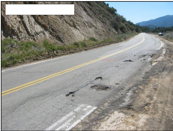
Figure 4.38: Preconstruction patching on 07-VEN-33.
