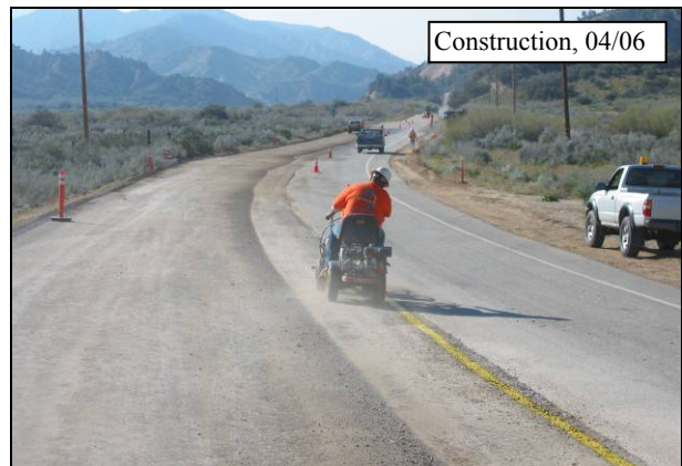
Figure 4.52: Temporary striping application on 07-VEN-33.
