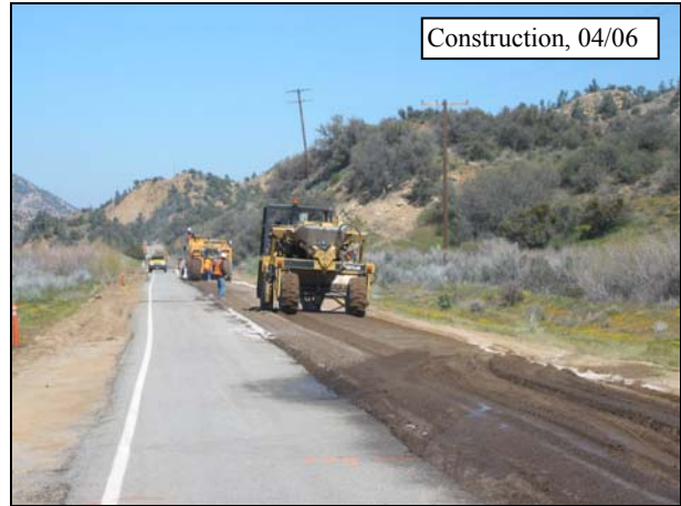
Figure 4.48: Water application behind recycling train on 07-VEN-33.
