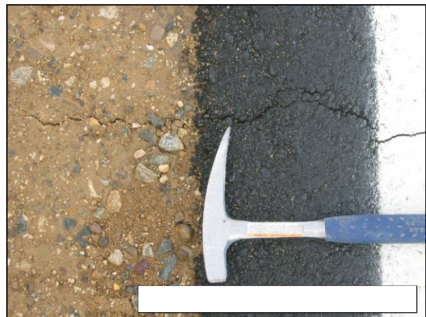
Figure 4.58: Transverse cracking on 07-VEN-33.
