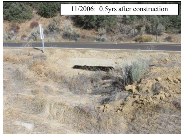
Figure 4.65: Blocked drain, including excess asphalt concrete from paving on 07-VEN-33. (2)
