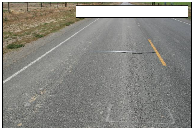
Figure 4.26: New areas of distress on 05-SB,SLO-33 (May 2008).
