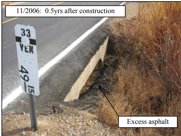
Figure 4.65: Blocked drain, including excess asphalt concrete from paving on 07-VEN-33. (2)
