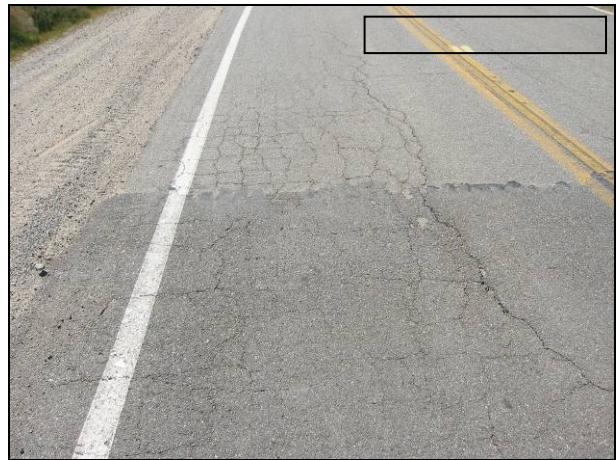
Figure 4.39: Preconstruction maintenance overlay on 07-VEN-33.
