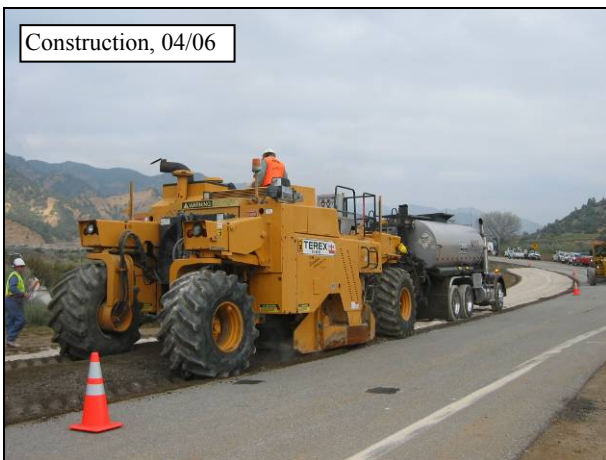
Figure 4.45: Foamed asphalt injection (Train 1) on 07-VEN-33.
