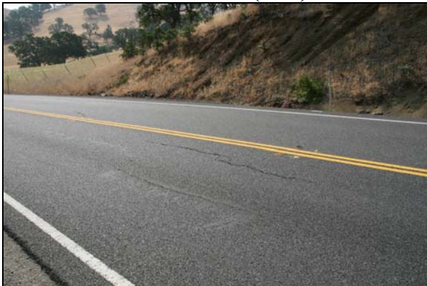
Figure 4.6: Longitudinal cracks in hill section on 03-COL-20 (2007–2008).
