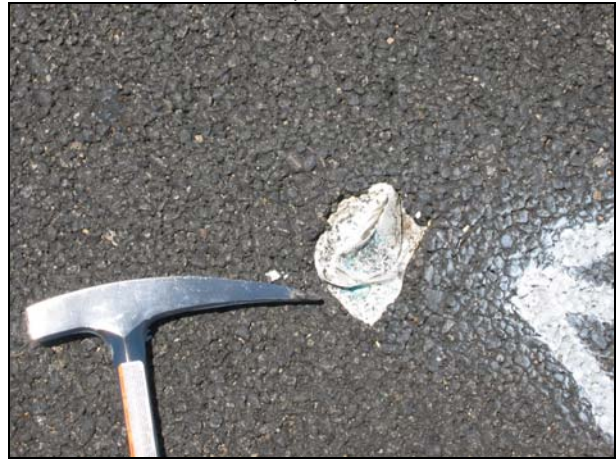
Figure 4.25: Trash compacted into asphalt concrete on 05-SB,SLO-33.
