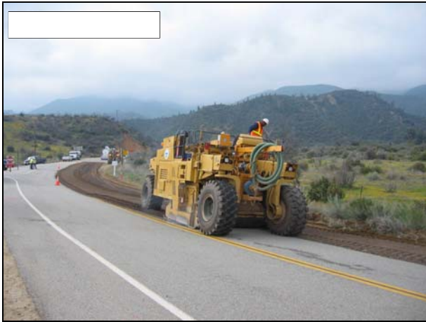
Figure 4.43: Prepulverization on on 07-VEN-33.
