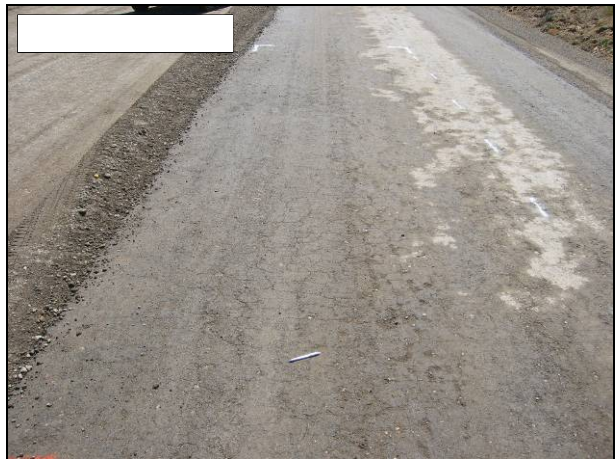
Figure 4.55: Area demarcated for rework on 07-VEN-33.
