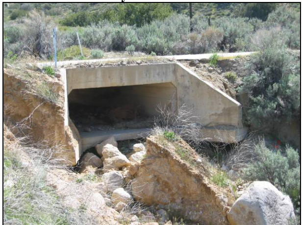
Figure 4.41: Drainage structure on 07-VEN-33.
