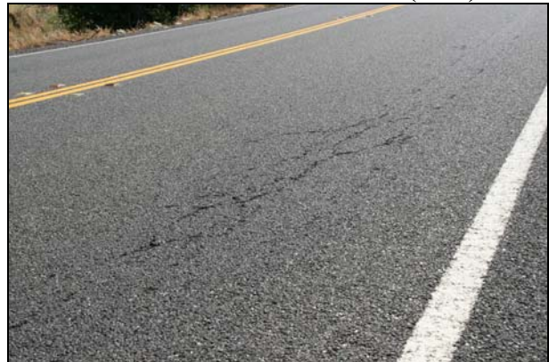
Figure 4.6: Longitudinal cracks in hill section on 03-COL-20 (2007–2008).
