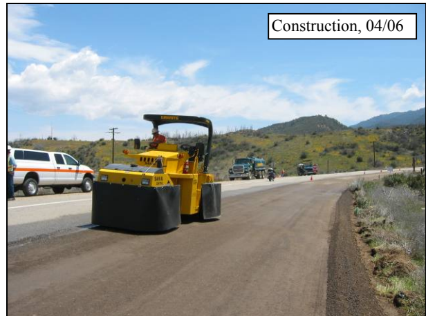
Figure 4.50: Final compaction with rubber-tired roller on 07-VEN-33.
