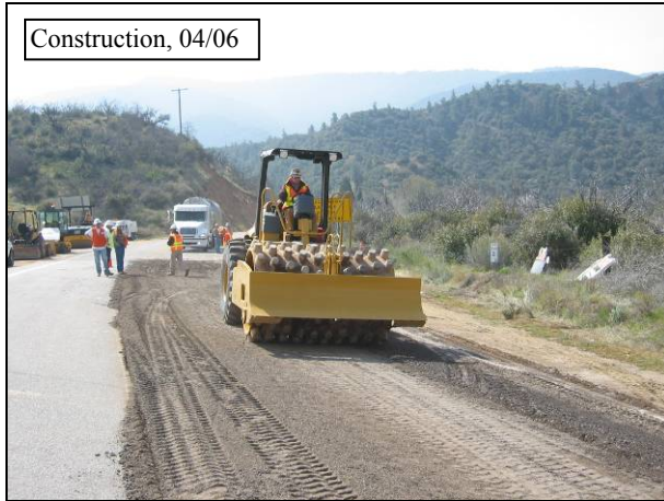
Figure 4.47: Initial compaction with padfoot roller on 07-VEN-33.
