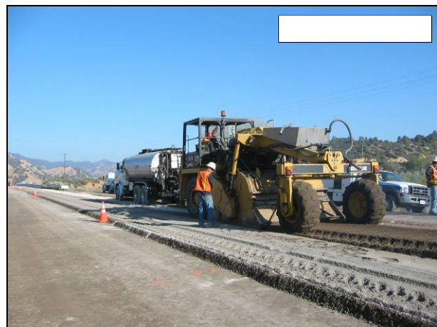
Figure 4.46: Foamed asphalt injection (Train 2) on 07-VEN-33.
