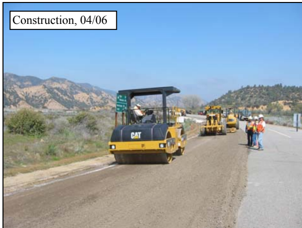
Figure 4.49: Shaping and compaction with steel wheel roller on 07-VEN-33.
