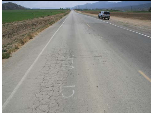
Figure 4.20: Proximity of irrigated fields to damaged road on 05-SB,SLO-33.
