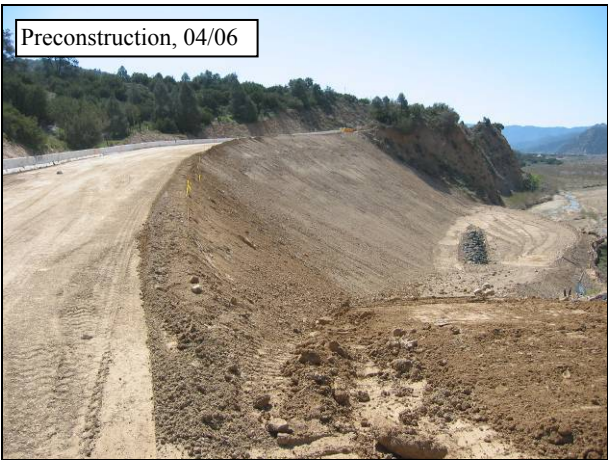
Figure 4.40: Pre-construction landslide repair on 07-VEN-33.
