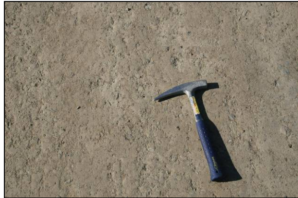
Figure 7.35: Good surface compaction in areas of recycling in normal temperatures.
