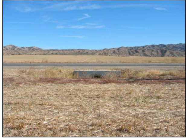
Figure 4.18: Filled in side drains on 05-SB,SLO-33.
