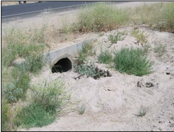
Figure 4.19: Blocked culvert on 05-SB,SLO-33.
