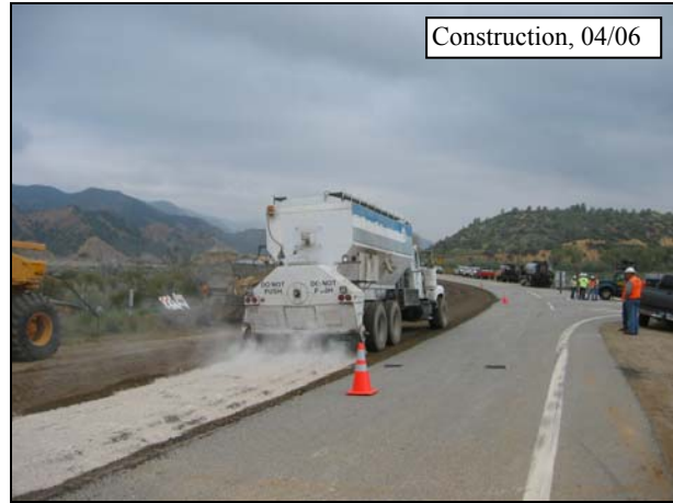
Figure 4.44: Cement kiln dust application on 07-VEN-33.
