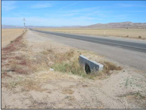
Figure 4.18: Filled in side drains on 05-SB,SLO-33.
