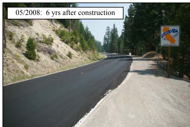
Figure 4.11: Pavement preservation treatment on 03-SIE-89.
