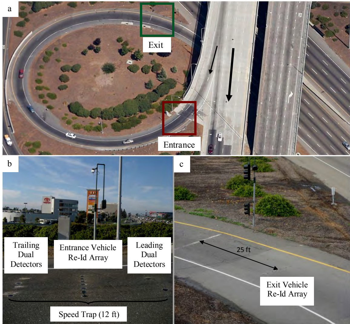
FIGURE 2 (a) Hegenberger on-ramp entrance and exit. (b) Vehicle detection system installation at the entrance of the ramp. (c) Sensor array installation at the exit of the ramp.
