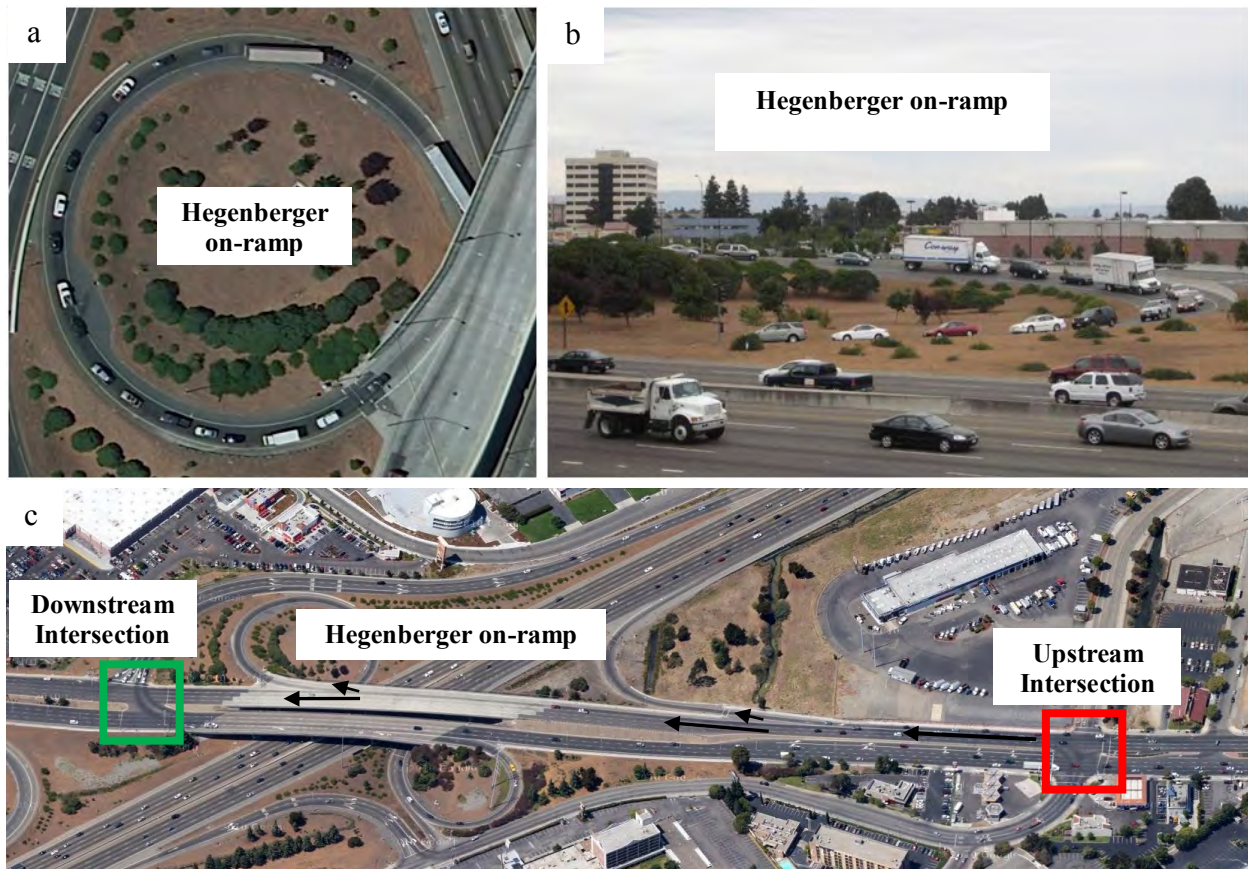
FIGURE 1 Hegenerberger on-ramp (a) aerial view with saturated queue, (b) side view with saturated queue and (c) arterial streets and intersections around the Hegenerberger on-ramp.
