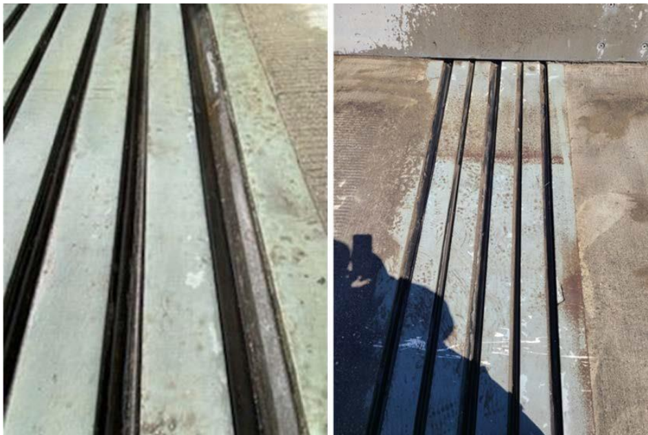
Figure 3.3: Bay Bridge joints after cleaning (Images from Caltrans District 4)
