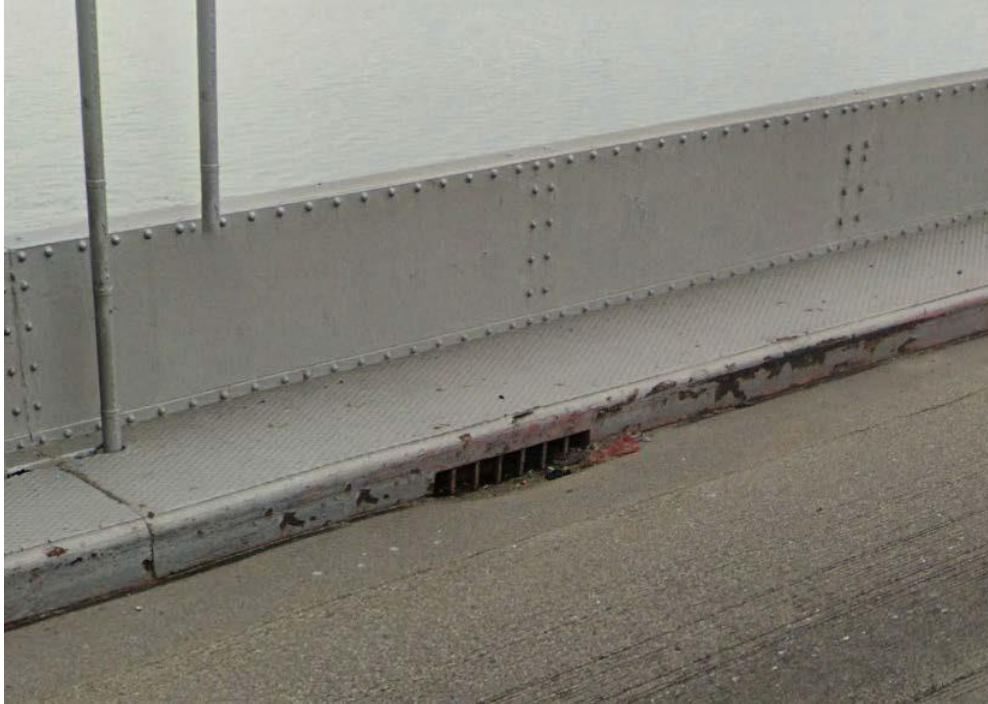
Figure 3.6: Scuppers (Google Street View image Dec 2020)
