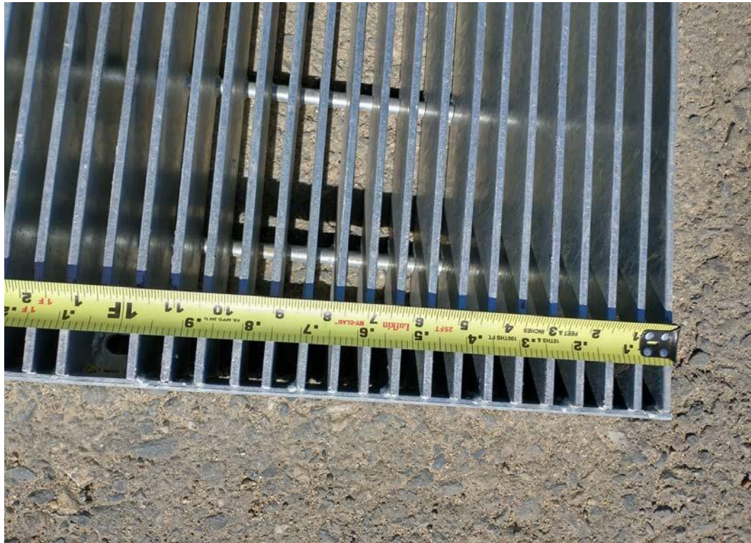
Figure 4.2: View of grate bottom
