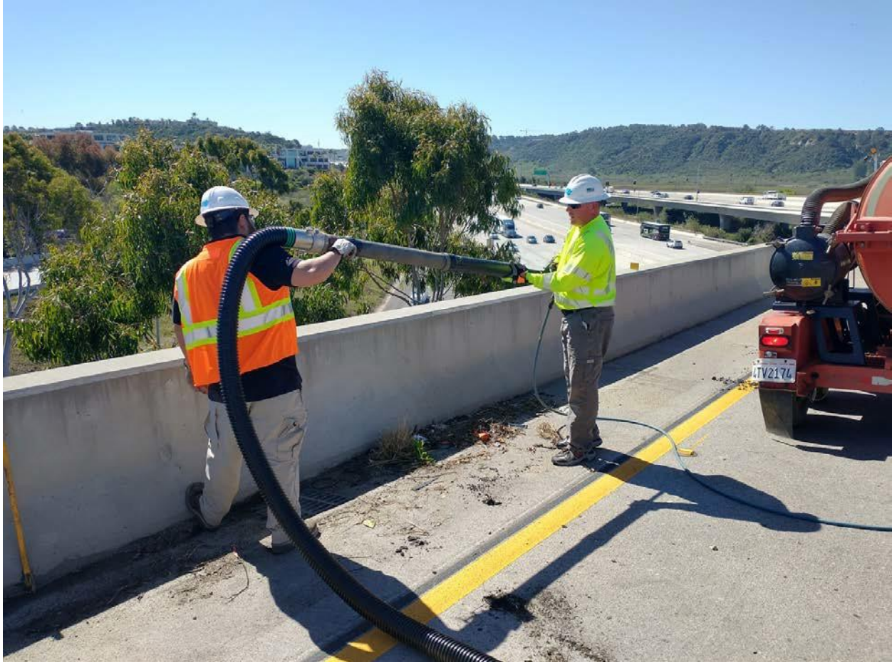
Figure 5.4: Clearing plugged hose
