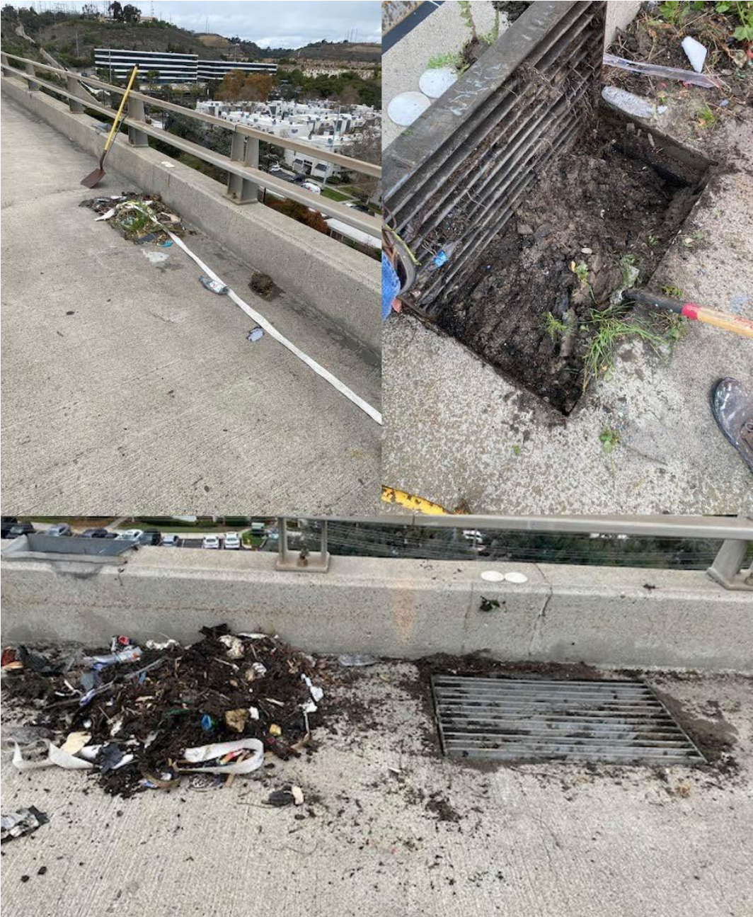
Figure 3.8: Example of drain cleaning on bridge in District 11 (Images from District 11)
