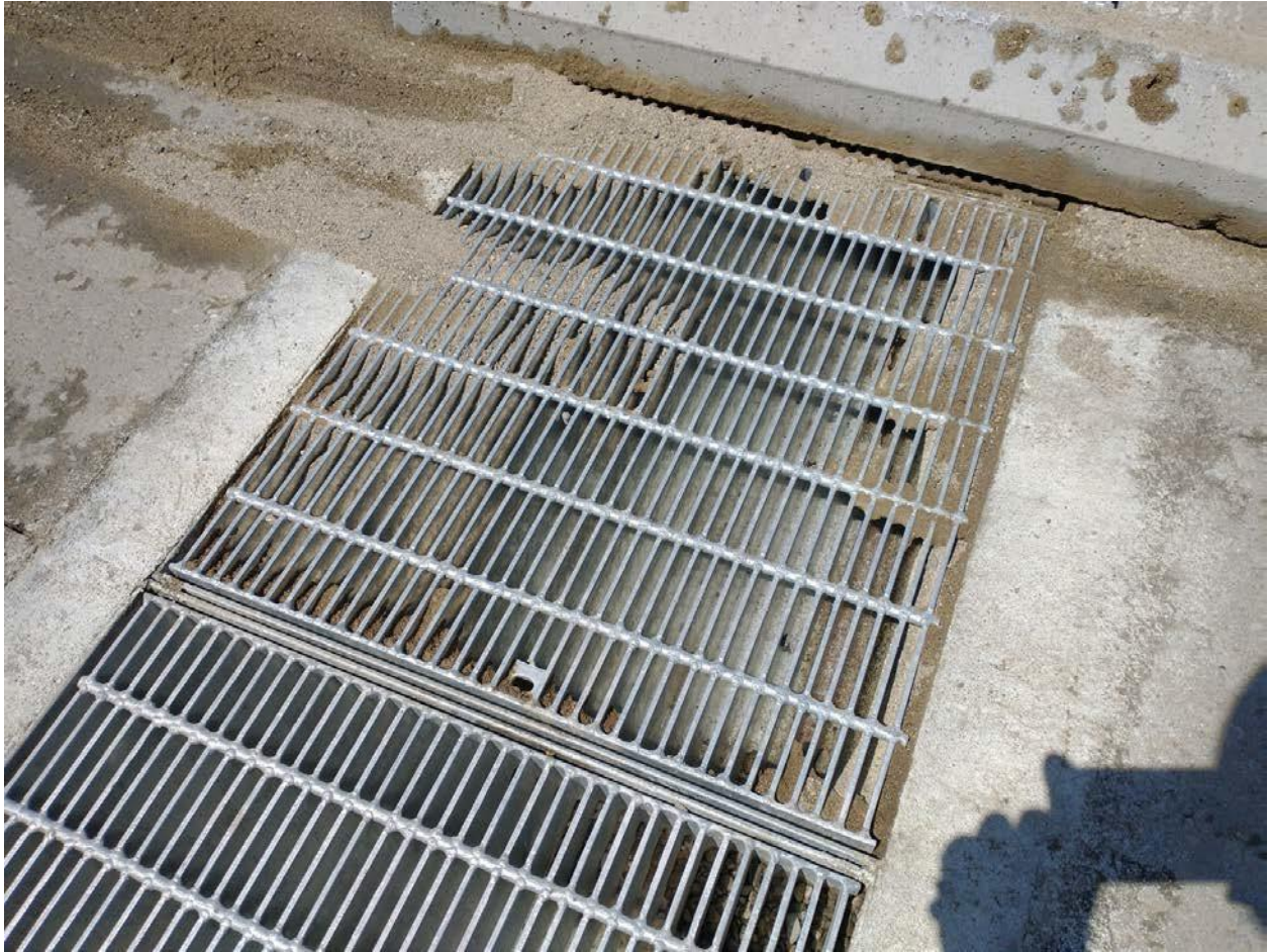
Figure B.6: Test#3 Pass 3 (sand after extensive stopextensive stopping)
