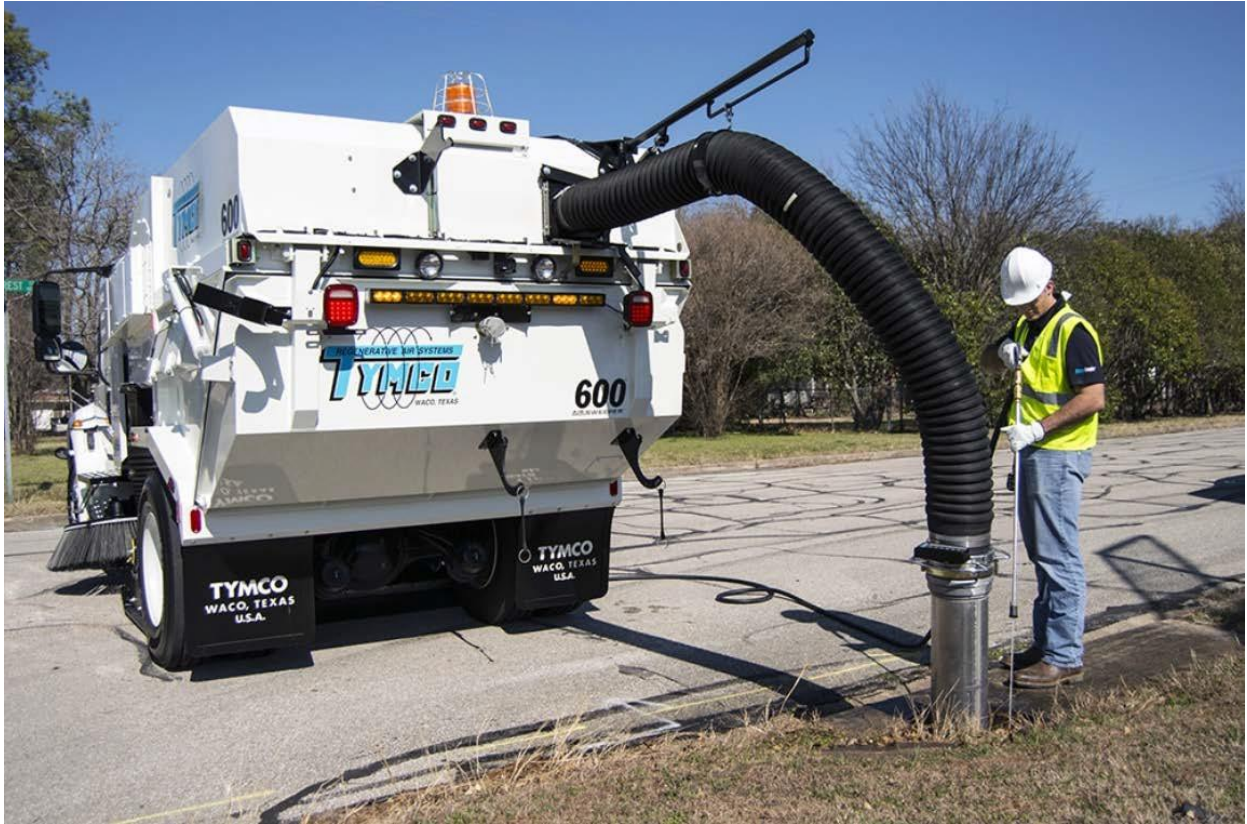
Figure 2.8: Catch basin cleaning using Tymco Regenerative Vacuum Sweeper 4 (Image from the Tymco website)
