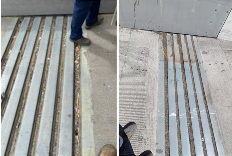
Figure 3.2: Bay Bridge joints before cleaning (Images from Caltrans District 4)
