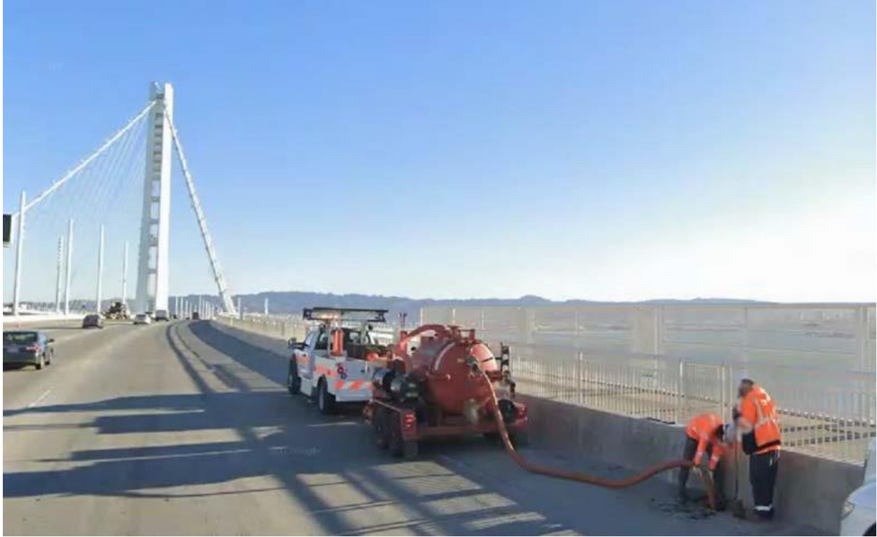
Figure 3.5: Drain cleaning on the Bay Bridge (Google Street View image Dec 2020)
