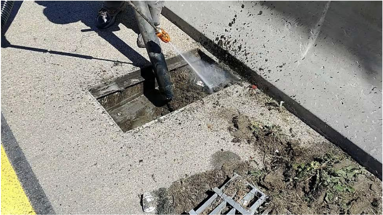
Figure 5.3: Cleaning with 3-in nozzle and swiveling power washer head
