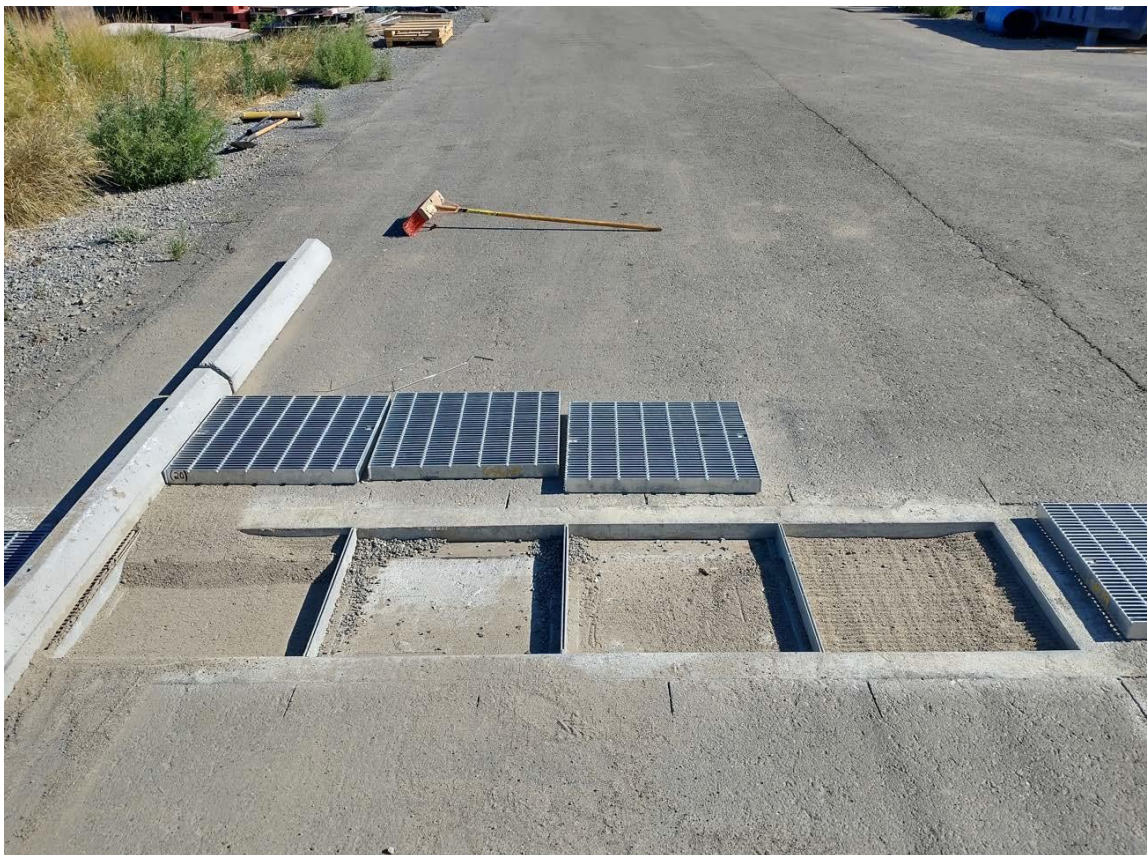
Figure 4.1: Installation of grates used to simulate an expansion joint at ATIRC
