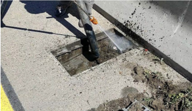
Image 2: Cleaning with a Ditch Witch 3-inch nozzle
