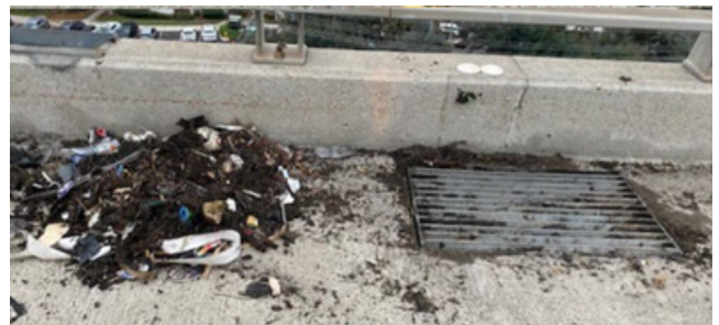
Image 1: Example of drain cleaning in District 11
