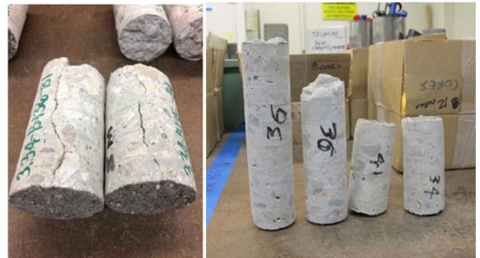
FIGURE 1: Bridge cores; cores equal to or longer than 3 inches were used for ASR visual inspection
